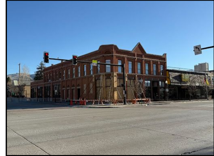
Maxwell Square Building. Photo courtesy of SHF Staff.
