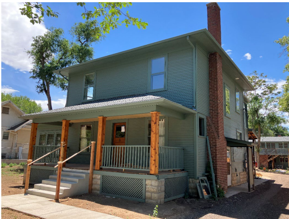
East and North facades
