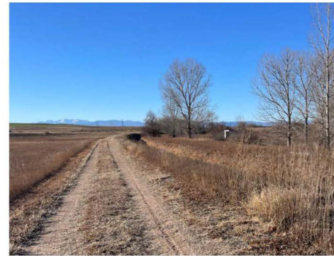
EXISTING DITCH ACCESS ROAD LOOKING WEST
