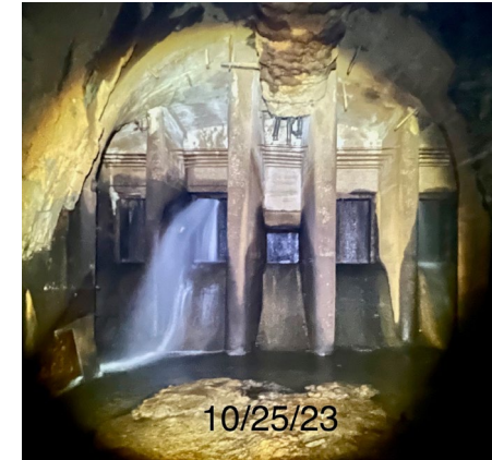
Milton Seaman Outlet Works $6 Million
