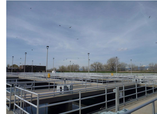
Boyd Flocculator Replacement $2 Million
