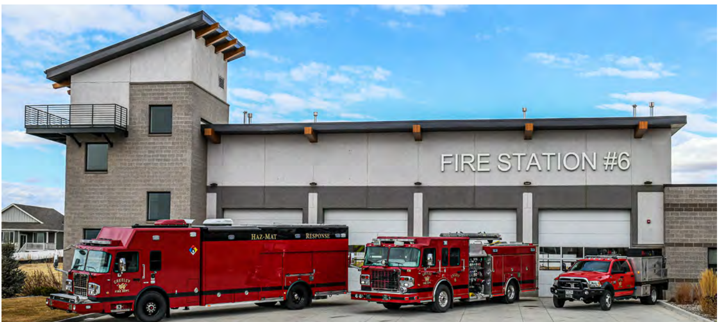
Fire Station 6 in Western Greeley
