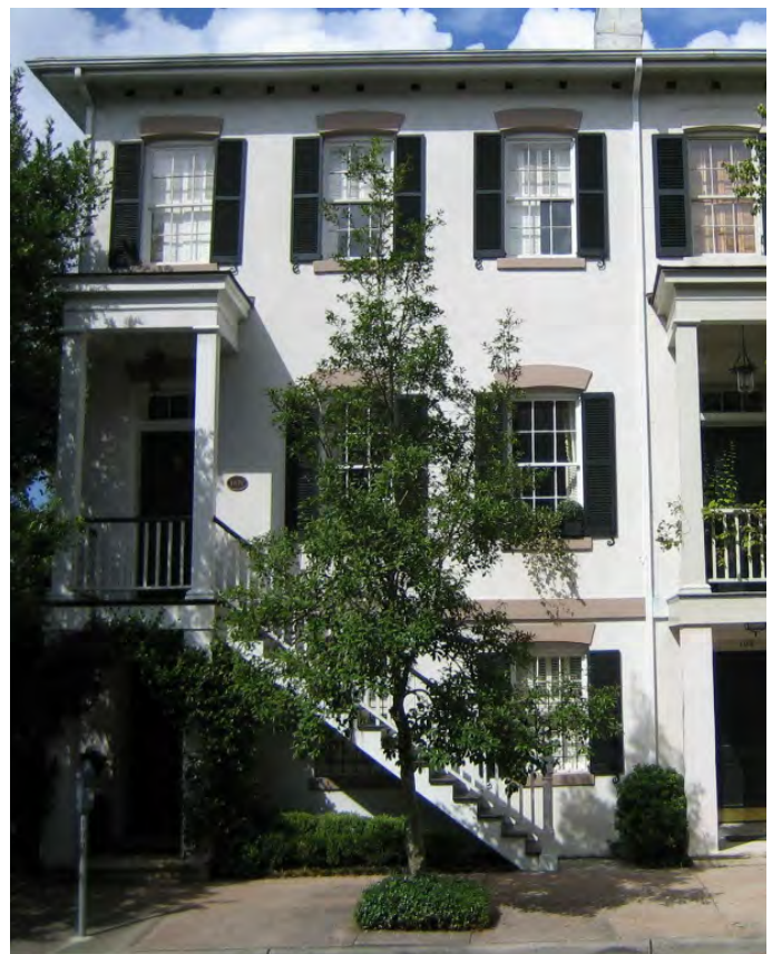
Figure 5-13: An at-grade entrance and an exterior stair leading to the entrance of the unit above.
