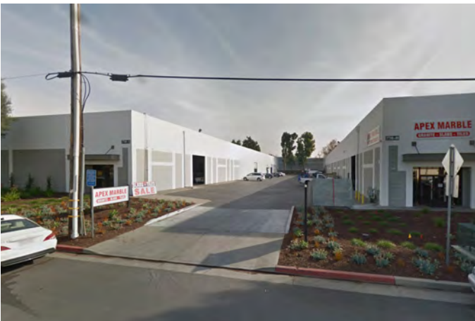
Industrial buildings and uses are also a part of the Workplace District.
