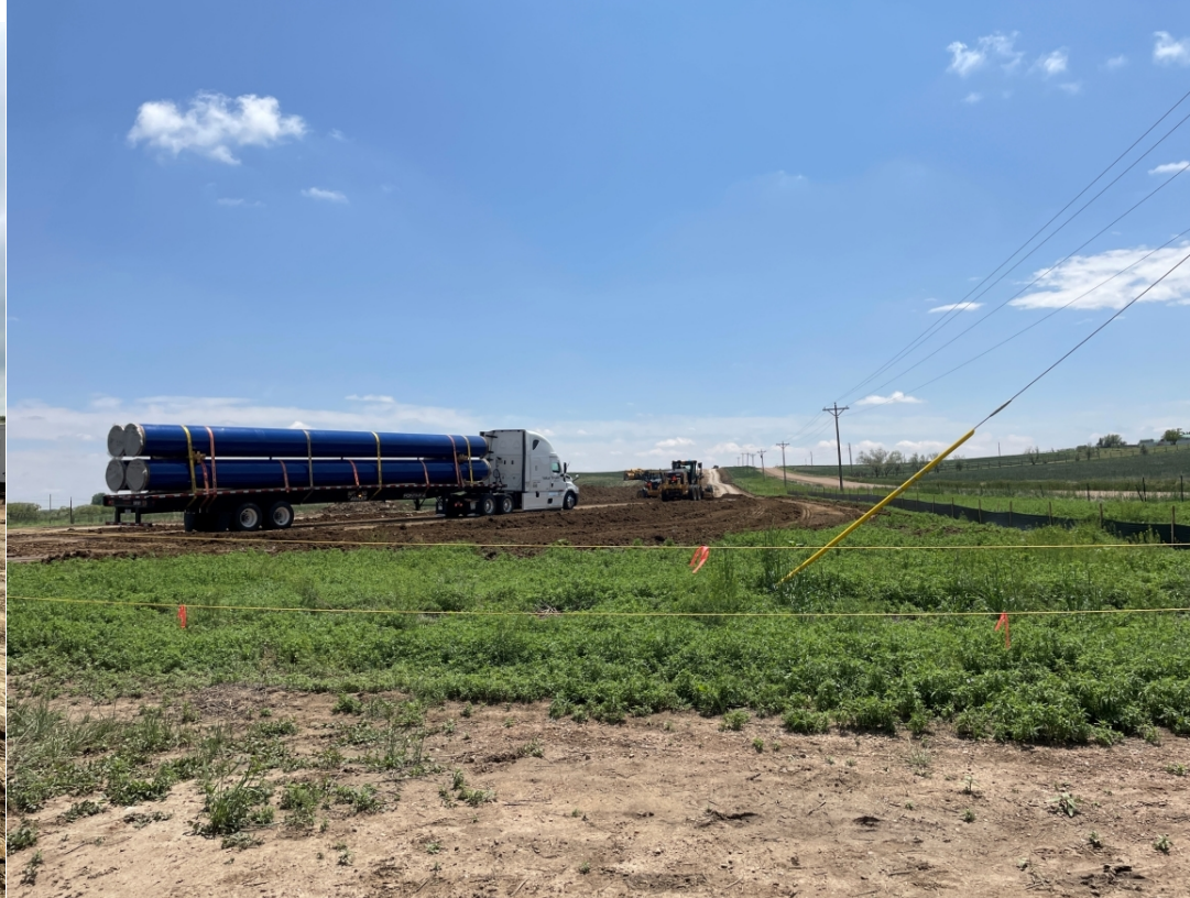
First loads of pipe arriving on site
