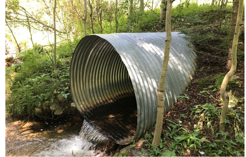
Perched culvert replaced with ford
