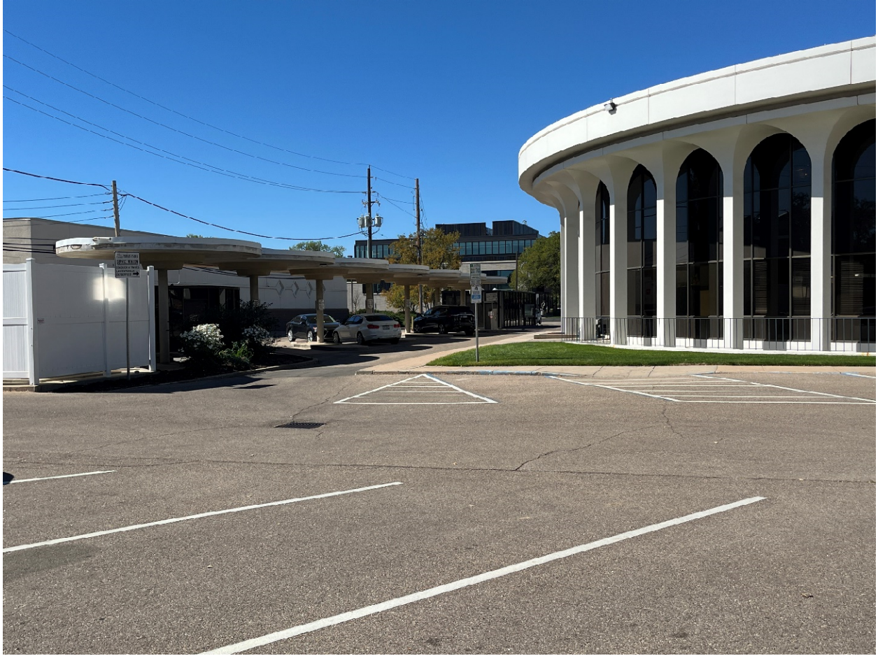
South façade and drive through bays south of the building
