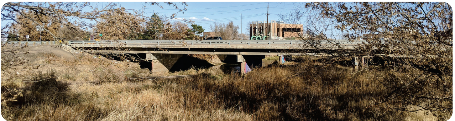
Figure 1. Kimley-Horn has long-standing relationships with the Lithos team and has most recently worked with them on the City's 12th Street Storm Outfall (Phase 1A) project (pictured below), for which they are providing tunneling expertise.
