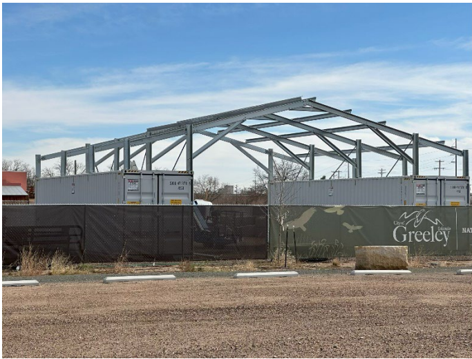
A new equipment shelter is being constructed in the NAT yard.
