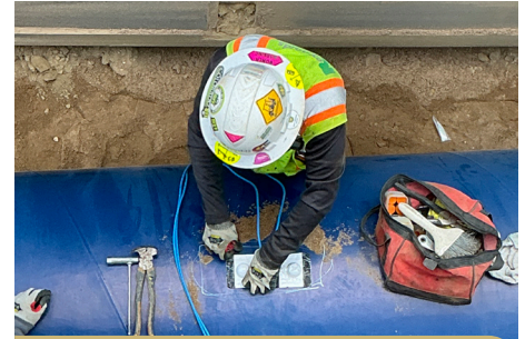
Installing Cathodic Protection on Watermain
