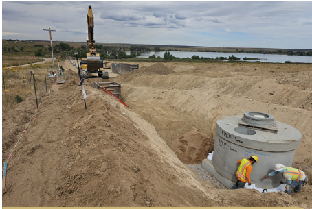
Backfilling Manhole for Combination Air Vacuum Valves
