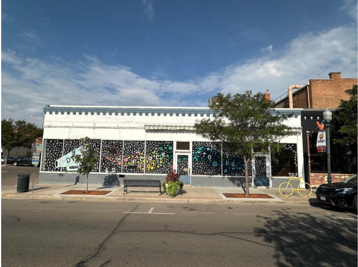
View of the east side of the entire building. The brick on the bottom of the building is currently painted grey, while the brick at the top of the building is painted white. ( View of photo is facing west ).
