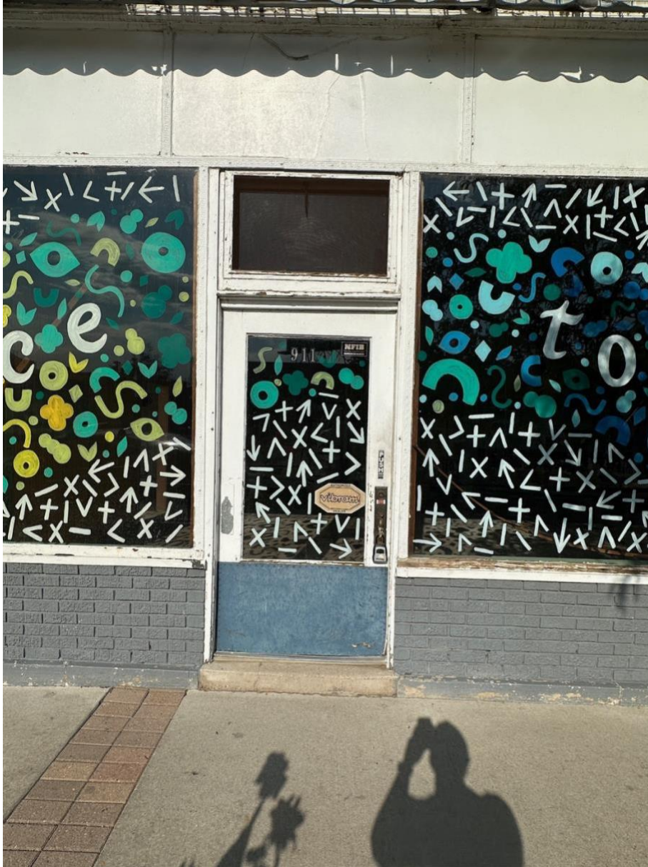
Existing south entrance on east side of building – this entrance will be closed off.
