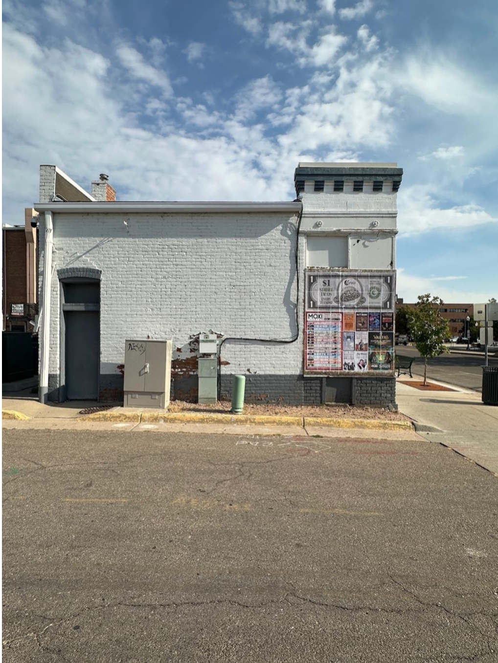
View of the entire south side of the building that faces the parking lot entrance. This is the proposed mural location. ( View of photo is facing north )
