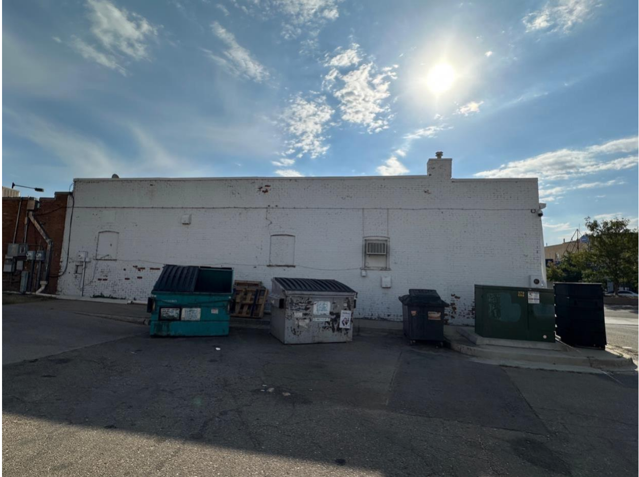
View of entire west face of the building, which faces the parking lot. Existing windows are boarded up but will be replaced. ( View of photo is facing east )
