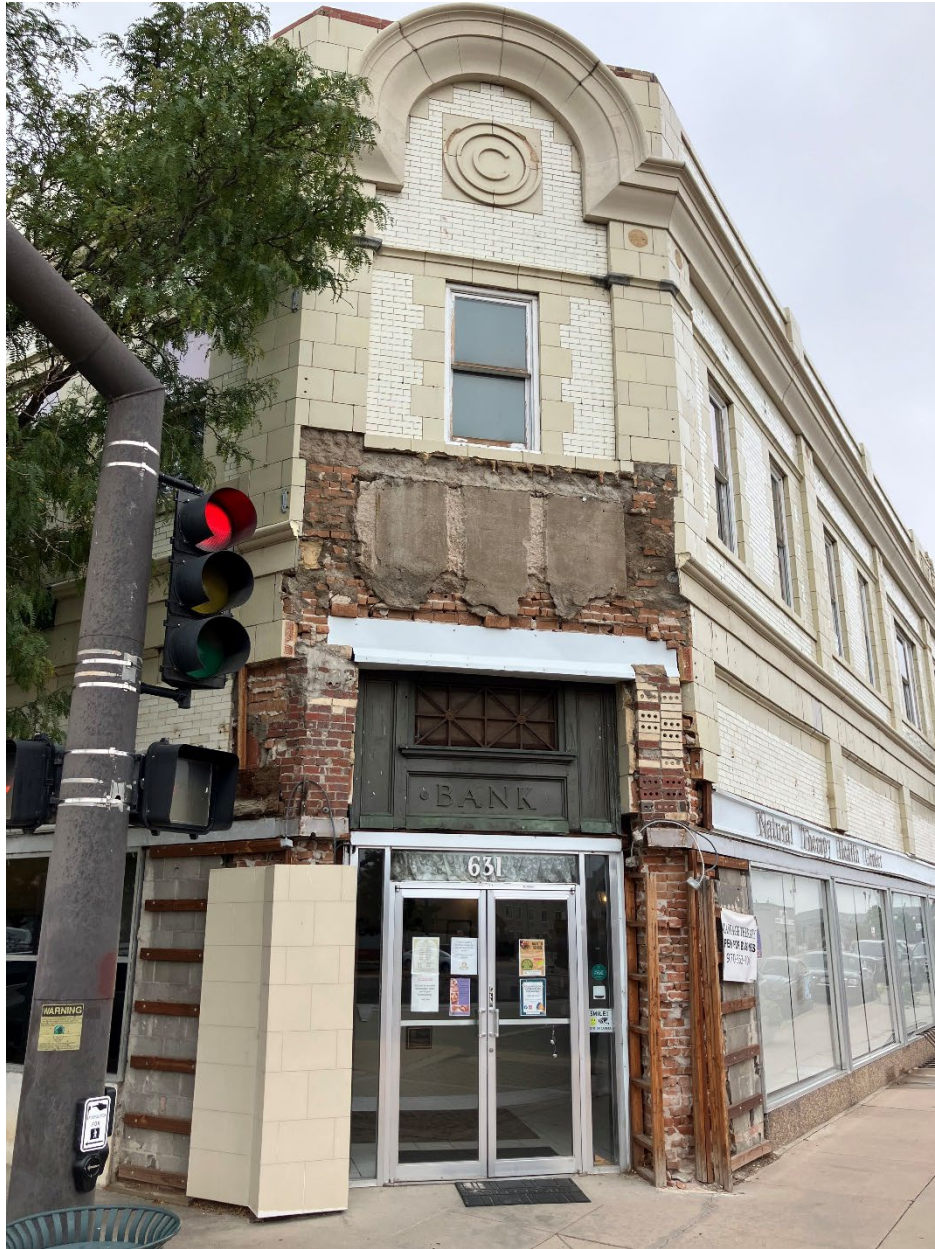
Southeast corner, view looking northwest
