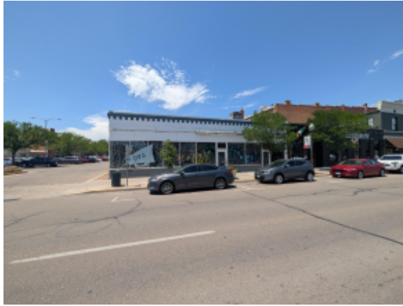
2 EXISTING EAST BUILDING IMAGE A5 N.T.S.
