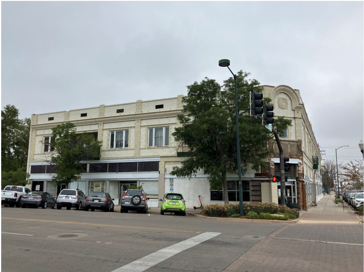
South façade; view looking north
