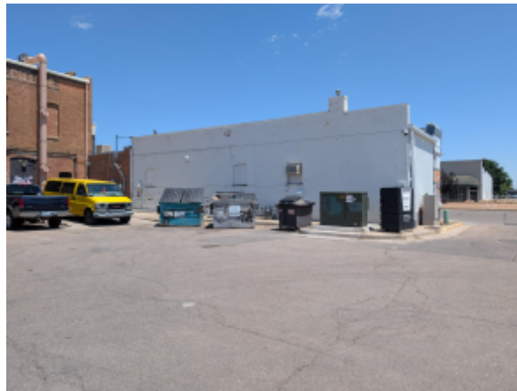
3 EXISTING WEST BUILDING IMAGE A5 N.T.S.
