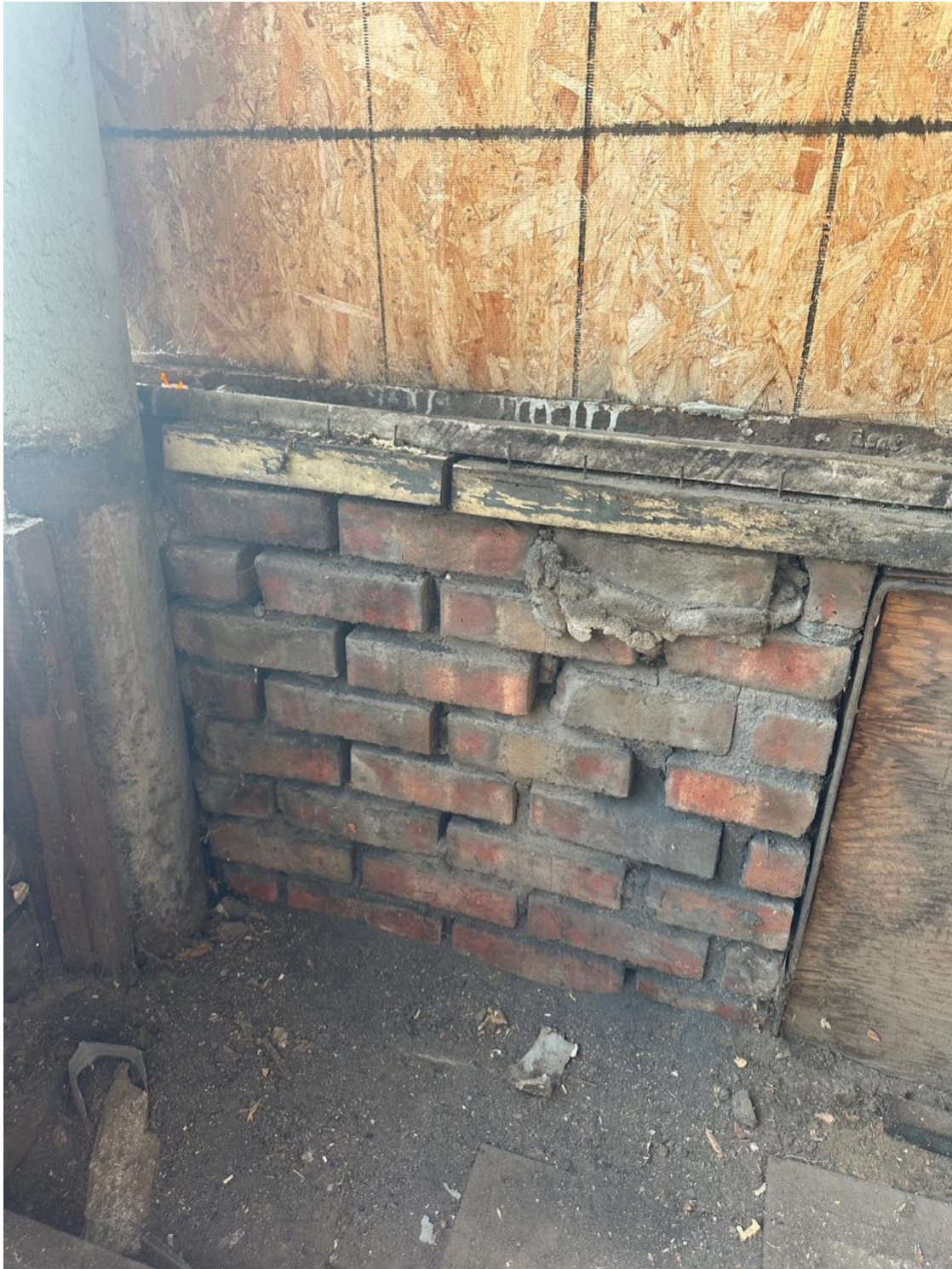
This is the interior of the SE corner of the building, showing the currently boarded up window that will be replaced and interior side of the brick. ( View of photo is facing south )
