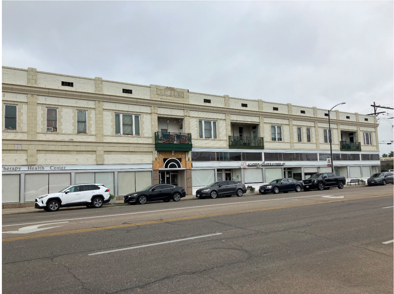
East façade, view looking west
