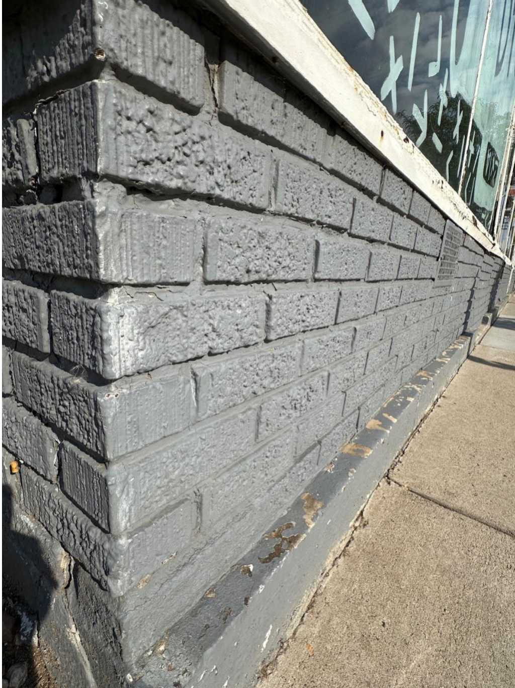
Close-up of existing painted brick on SE corner of building. Brick will be repainted. ( View of photo is facing NW )
