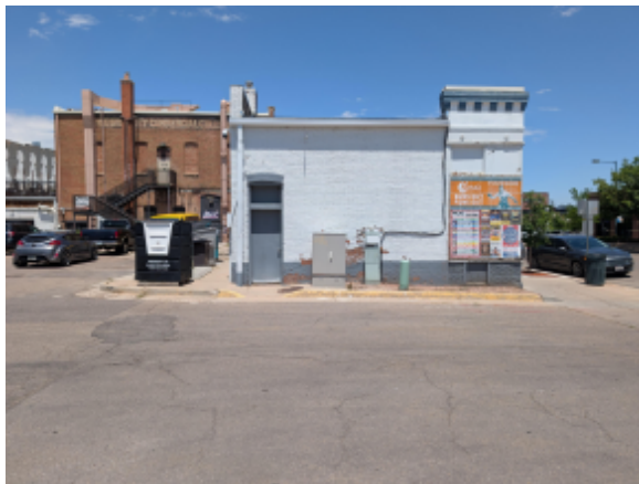
4 EXISTING SOUTH BUILDING IMAGE A5 N.T.S.
