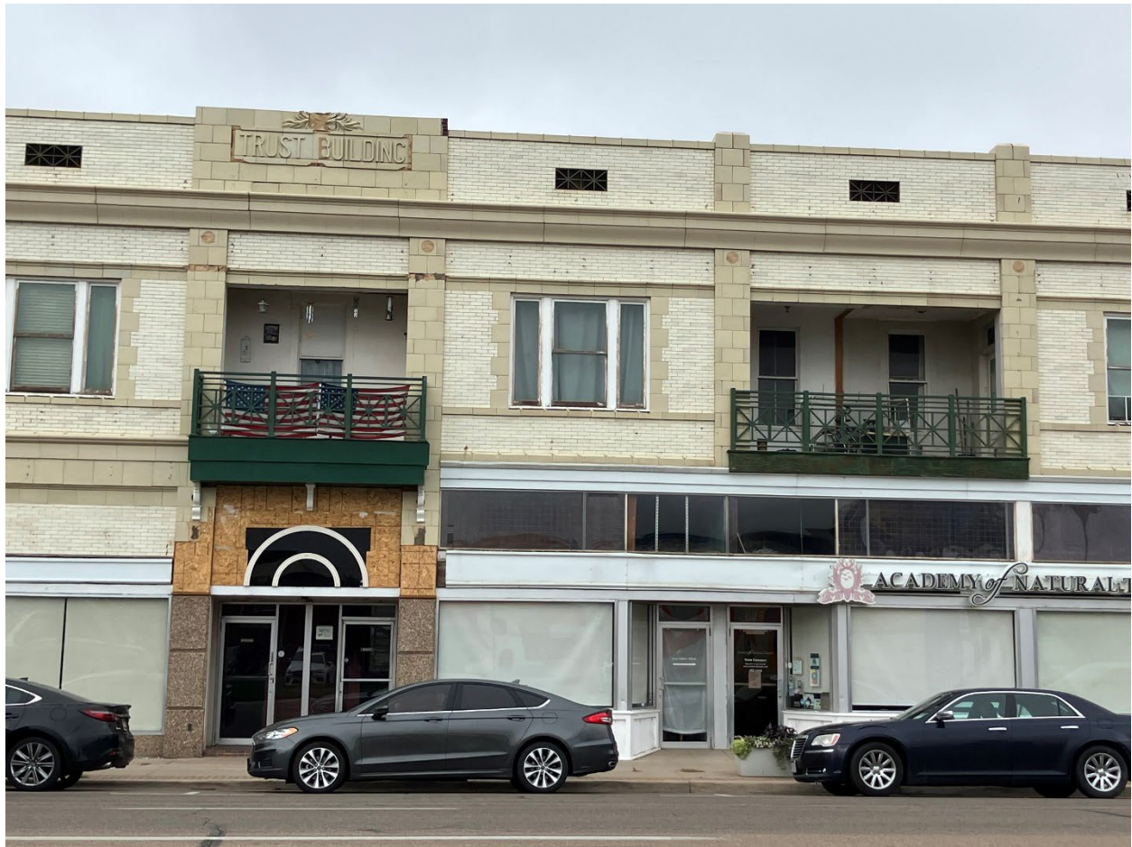
8 th Avenue entrances on east façade, view looking west
