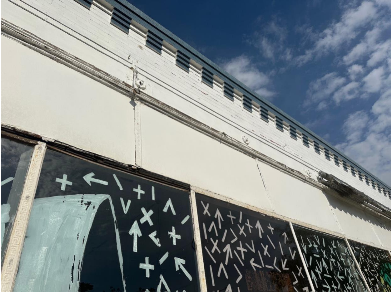
Another view showing the upper painted windows, flower design, and roofline. The awning on the right side of the photo will be removed, as it is unsalvageable. ( View of photo is facing west )
