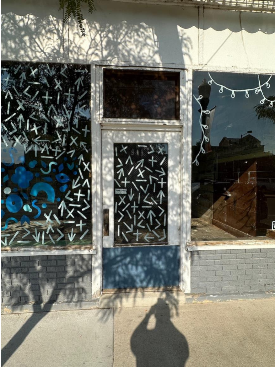
Existing north entrance on east side of building – this is the entrance that will be inset and widened to accommodate ACA.
