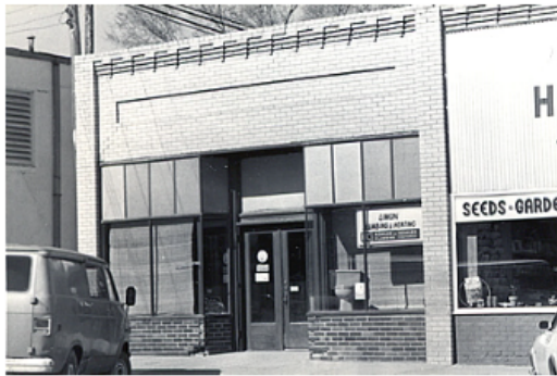
An example of the early twentieth-century commercial special use types on E Avenue in Limon.
