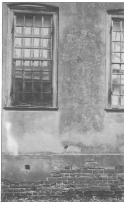
Excessive moisture has damaged not only the stuccoed wall surface, but also the brick substrate.
