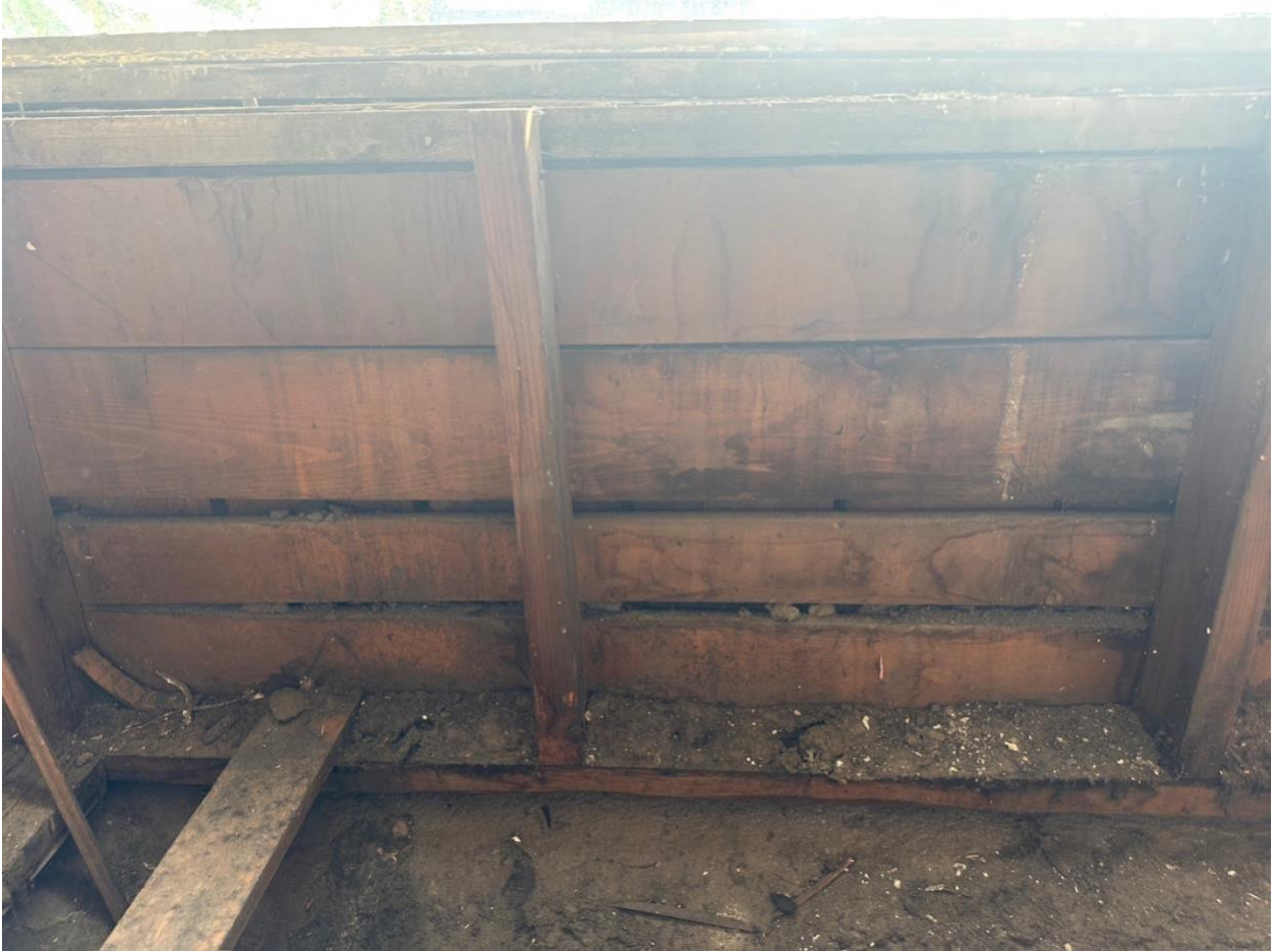
This is the interior of the building below the storefront windows. ( View of photo is facing east )
