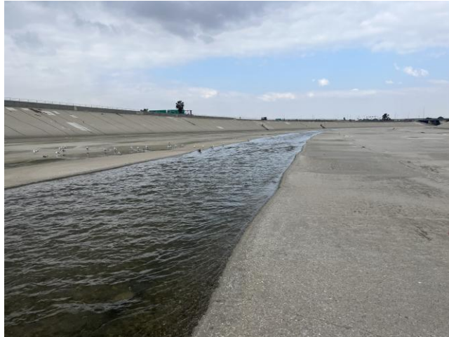
Figure 2 Tall levees along the LA river, designed to protect infrastructure from flooding, discourage access.
