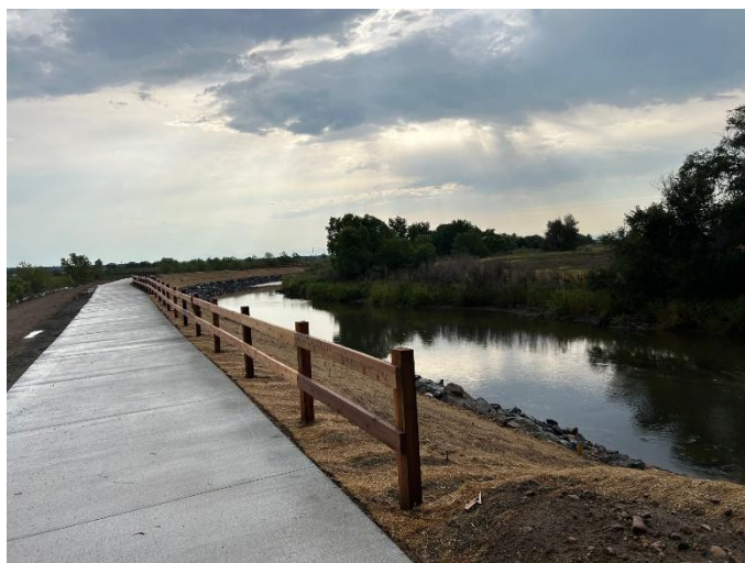
View to the west of the completed Poudre Ponds river restoration project.
