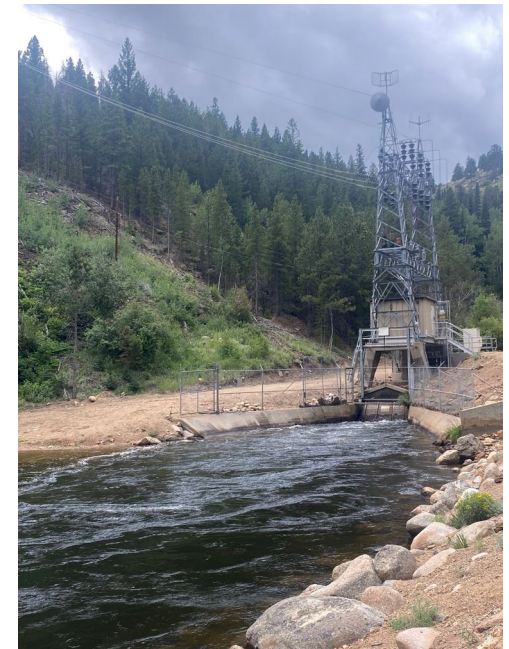
Adams Tunnel Outlet – Larimer Co
