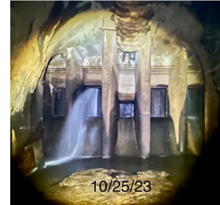
Milton Seaman Outlet Works $6 Million
