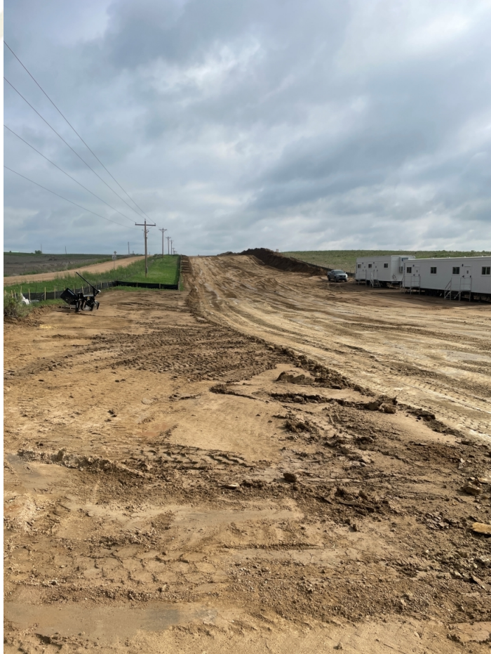
Segment 2 ROW prepped for pipe
