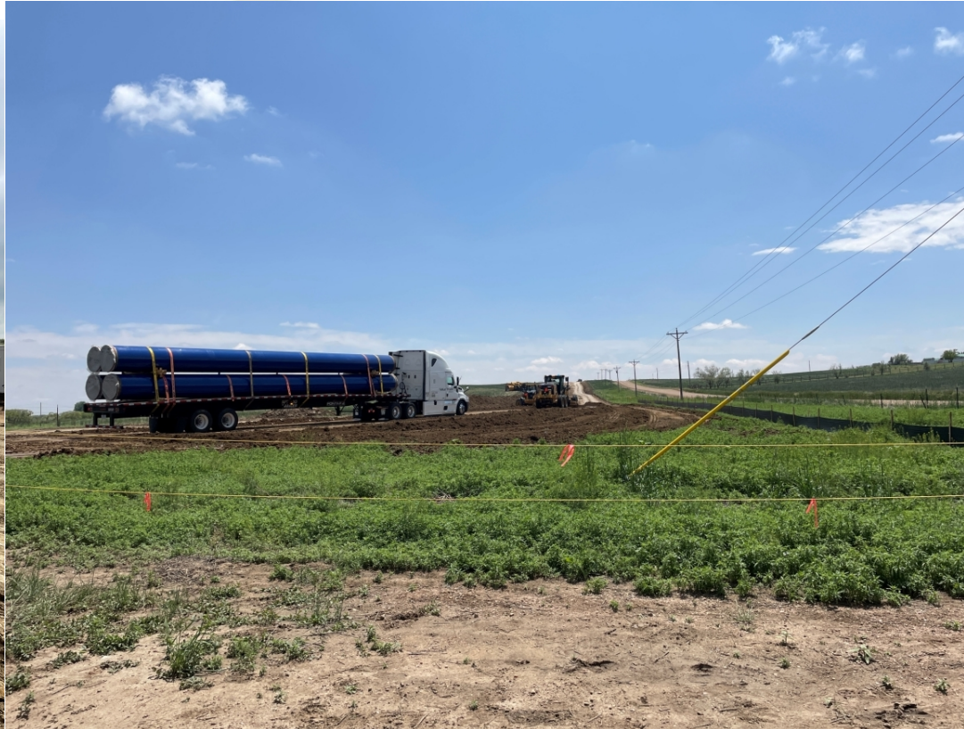
First loads of pipe arriving on site
