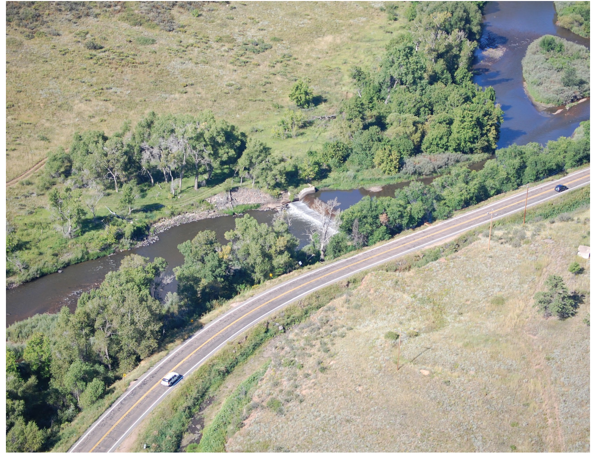
Poudre River Diversion
