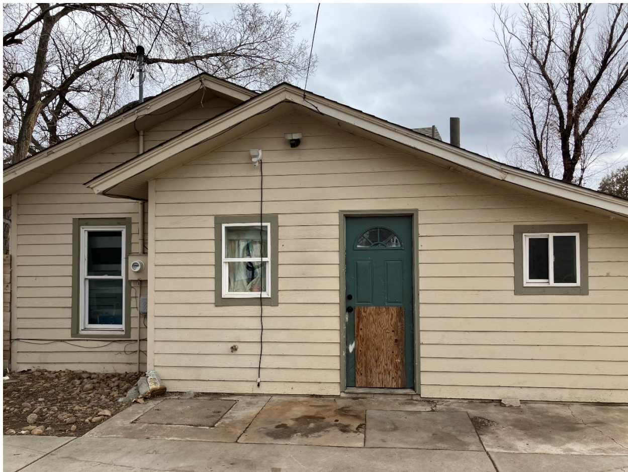
North façade, March 2025, photo by Betsy Kellums, GHPO
