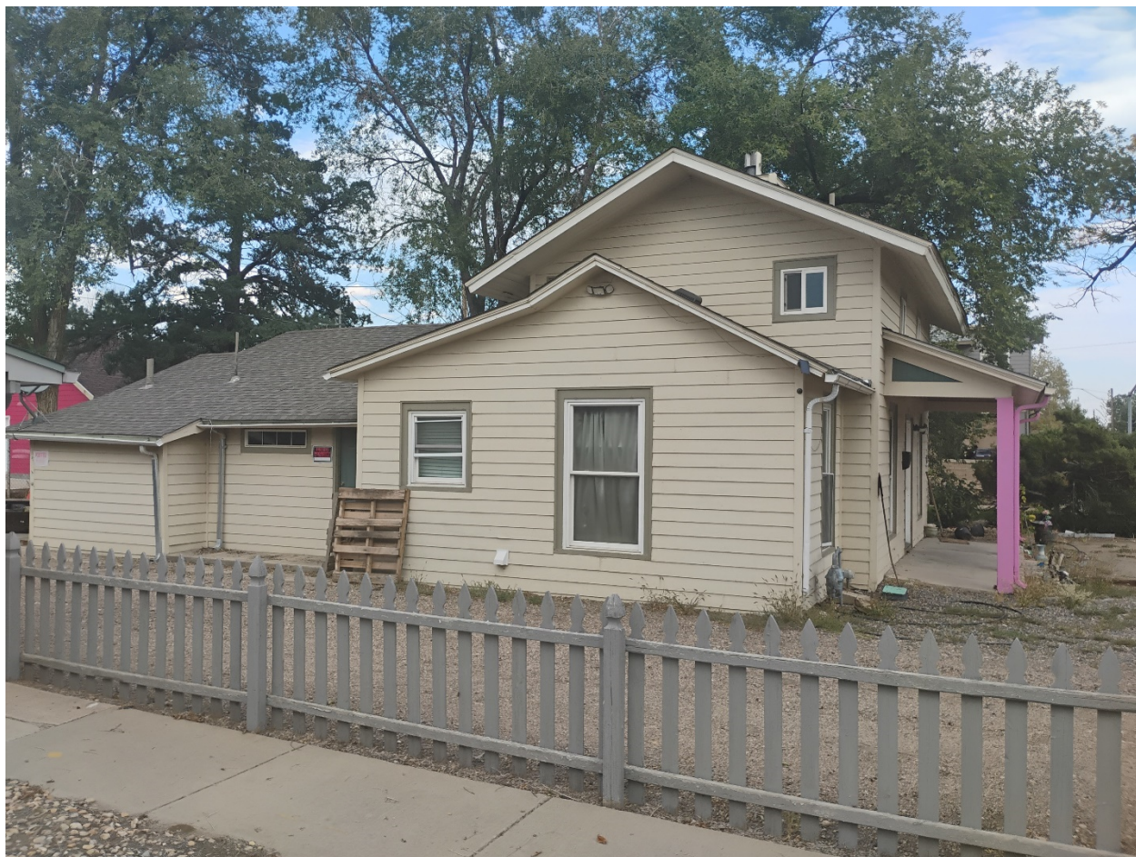
West façade, January 2025, photo by owner Jason Pressley
