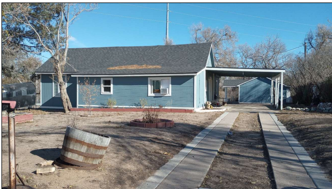
Site 5WL9808. Overview of the property from 23 rd Avenue, facing east. Photo by E. Garner, 11/19/2024.
