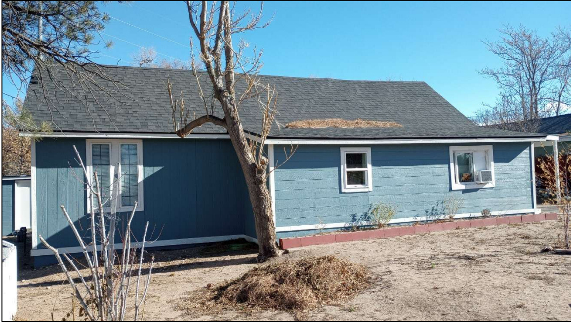
Site 5WL9808. The west elevation of Feature 1 (1943 residence) capturing the west and north additions, facing southeast. Photo by E. Garner, 11/19/2024.
