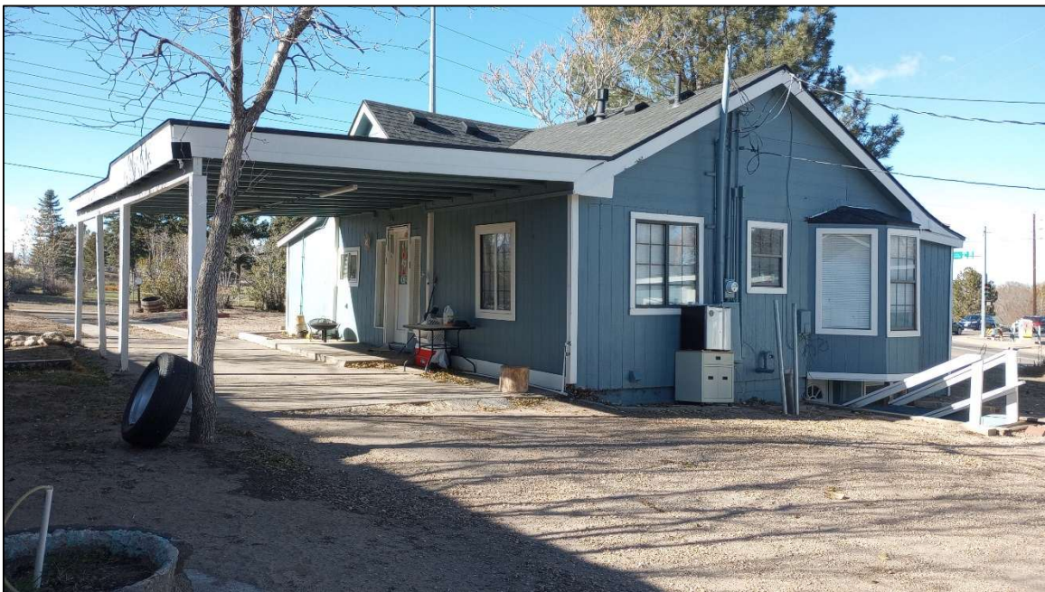
Site 5WL9808. The south façade, carport, and east elevation of the east addition of Feature 1 (1943 residence), facing northwest. Photo by E. Garner, 11/19/2024.
