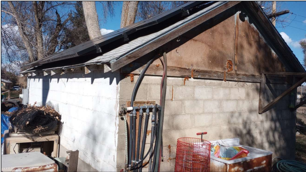
Site 5WL9807. The west and south elevations of Feature 2 (1952 garage), facing northeast. Photo by E. Garner, 11/19/2024.
