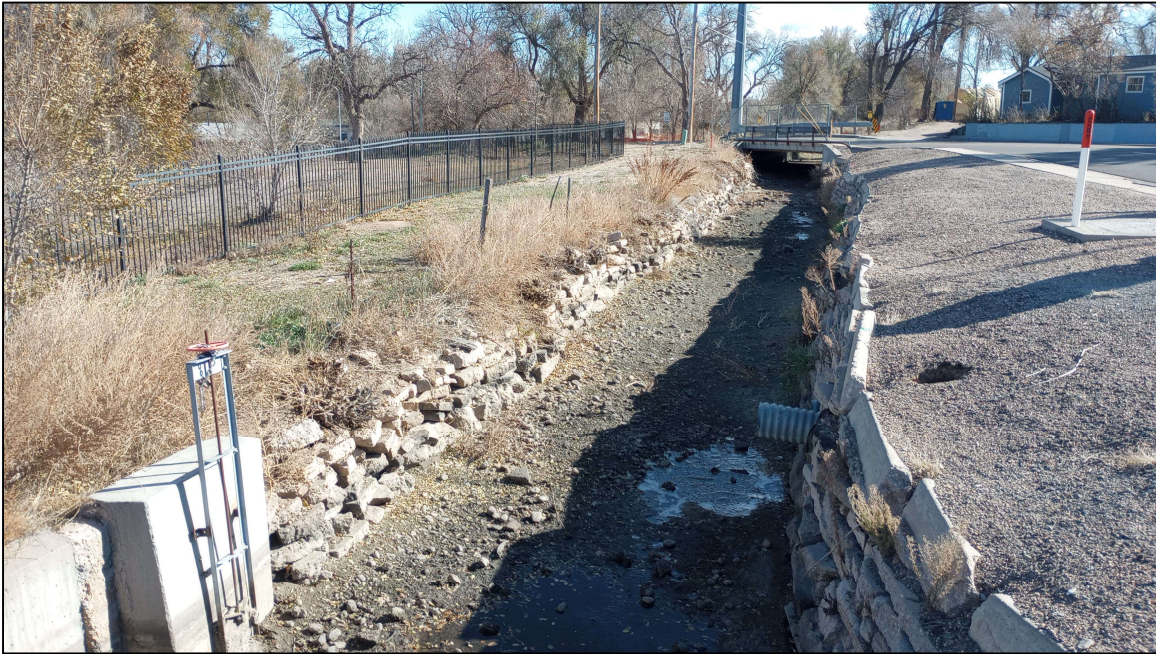
Site 5WL843.20. Overview of ditch from northwest end of segment, facing southeast. Feature 1 visible in the left foreground and the 5 th Street bridge visible in background. E. Garner, 11/19/2024.
