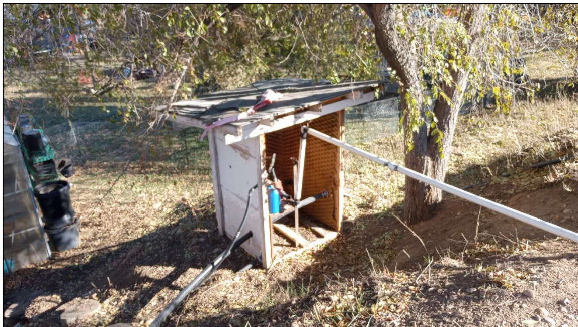
Site 5WL9807. The north elevation and the interior of Feature 4 (pumphouse), facing southeast. Photo by E. Garner, 11/19/2024.
