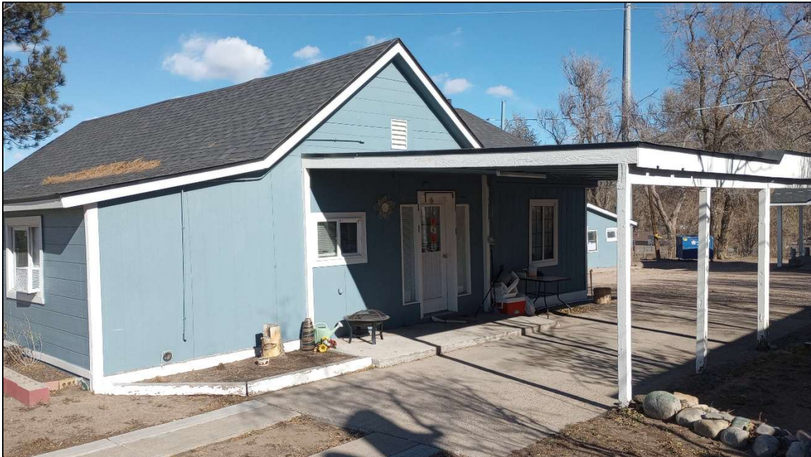
Site 5WL9808. The south-facing façade with carport of Feature 1 (1943 residence), facing northeast. Photo by E. Garner, 11/19/2024.
