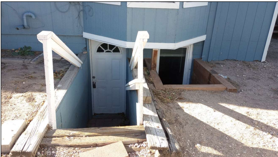
Site 5WL9808. Entrance to the basement apartment on the east elevation of Feature 1 (1943 residence) facing west. Photo by E. Garner, 11/19/2024.
