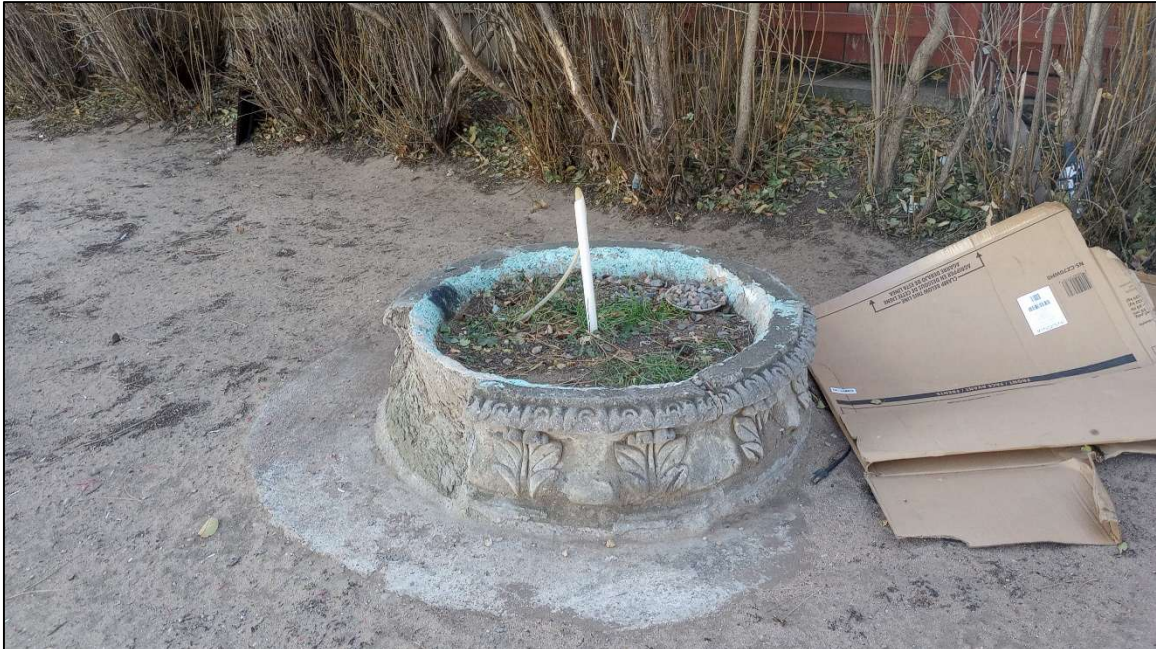
Site 5WL9808. Overview of Feature 5 (possible cistern), facing southeast. Photo by E. Garner, 11/19/2024.
