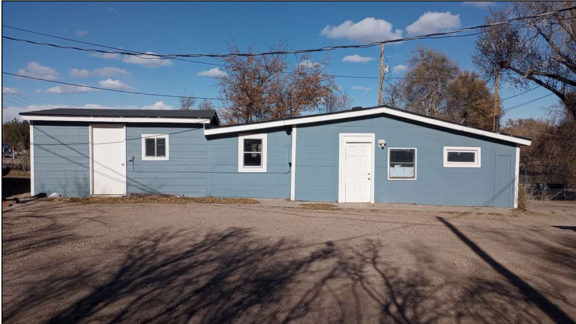
Site 5WL9808. The south-facing façade of Feature 2 (1943 converted garage) showing the east, central, and west additions, facing north. Photo by E. Garner, 11/19/2024.
