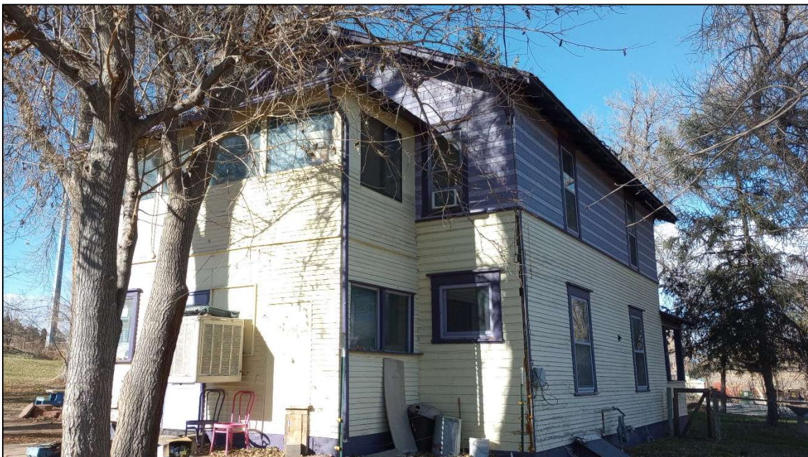
Site 5WL9807. The south and east elevations of Feature 1 (1899 residence), facing northwest. Photo by E. Garner, 11/19/2024.
