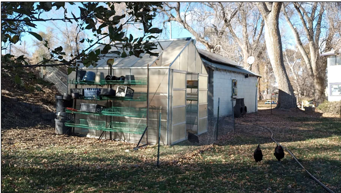
Site 5WL9807. The south and east elevations of Feature 3 (greenhouse) and the east elevation of Feature 2 (1952 garage), facing north-northwest. Photo by E. Garner, 11/19/2024.
