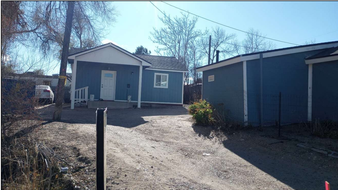
Site 5WL9808. Site overview showing the east part of the property and the north elevation of Feature 3 (1999 residence). Photo by E. Garner, 11/19/2024.
