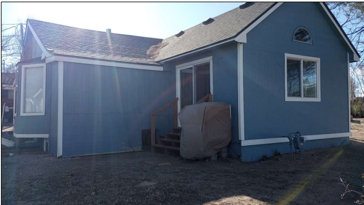
Site 5WL9808. The east and north elevations of the north addition and the north and east elevations of the east addition of Feature 1 (1943 residence), facing southwest. Photo by E. Garner, 11/19/2024.
