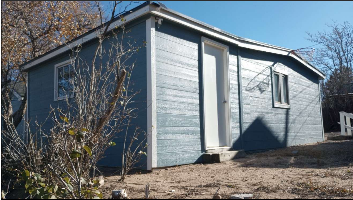
Site 5WL9808. The west and north elevations of Feature 2 (1943 converted garage) highlighting the west and northwest additions, facing southeast. Photo by E. Garner, 11/19/2024.
