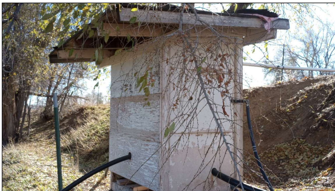
Site 5WL9807. The east and north elevations of Feature 4 (pumphouse), facing southwest. Photo by E. Garner, 11/19/2024.
