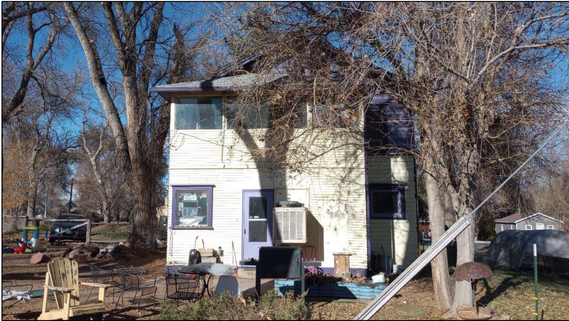
Site 5WL9807. The south elevation of Feature 1 (1899 residence) capturing the home addition, facing north. Photo by E. Garner, 11/19/2024.
