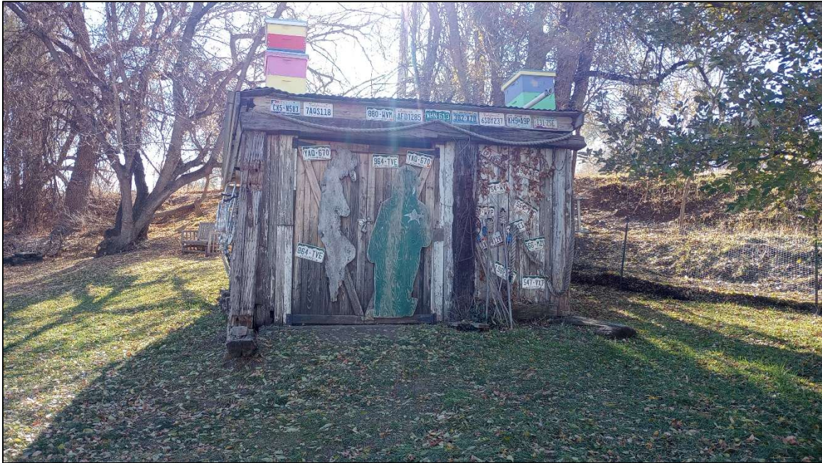
Site 5WL9807. The north elevation of Feature 5 (work shed), facing south. Photo by E. Garner, 11/19/2024.
