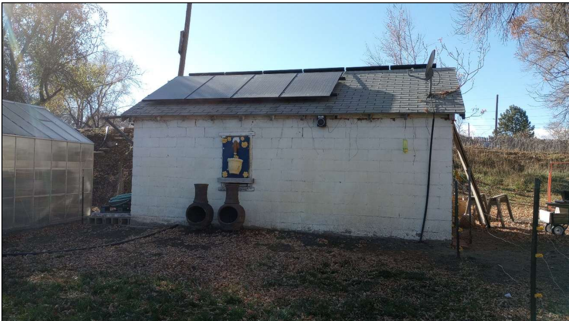
Site 5WL9807. The east elevation of Feature 2 (1952 garage) and the north elevation of Feature 3 (greenhouse), facing west. Photo by E. Garner, 11/19/2024.
