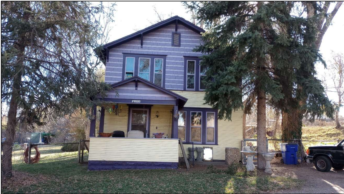
Site 5WL9807. The north-facing façade of Feature 1 (1899 residence), facing south. Photo by E. Garner, 11/19/2024.
