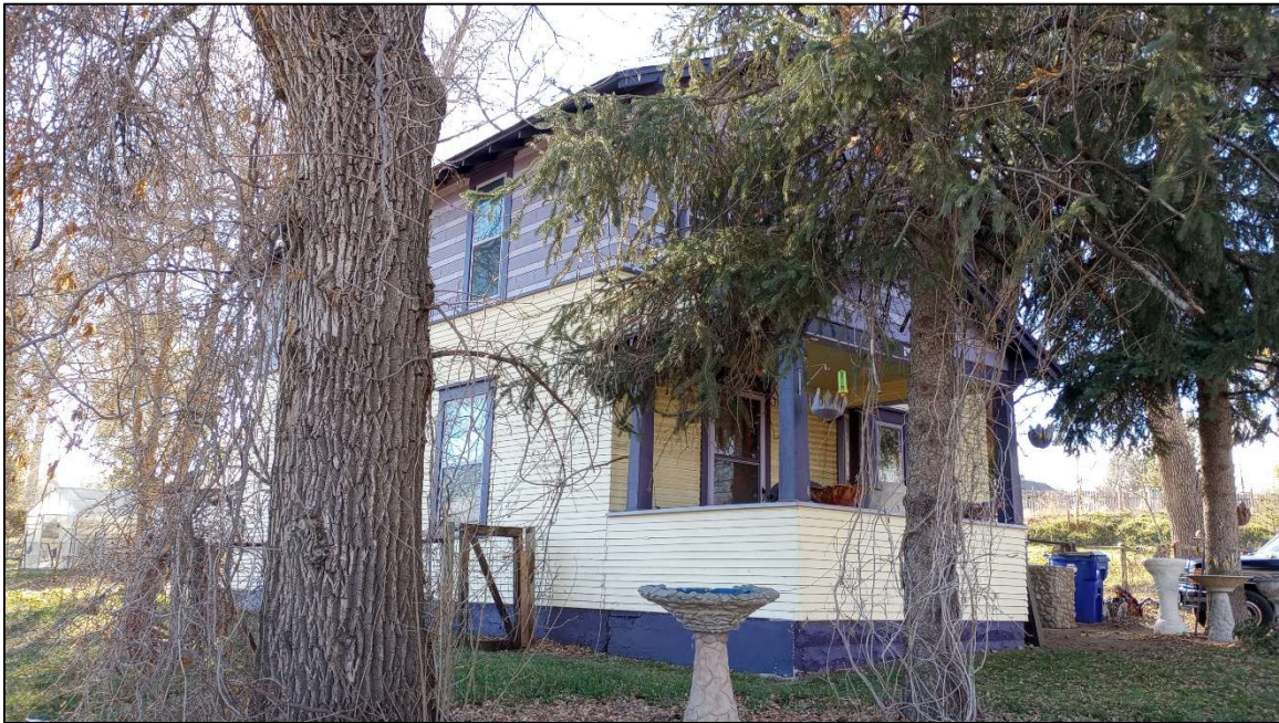
Site 5WL9807. The east and north elevations of Feature 1 (1899 residence,) facing southwest. Photo by E. Garner, 11/19/2024.
