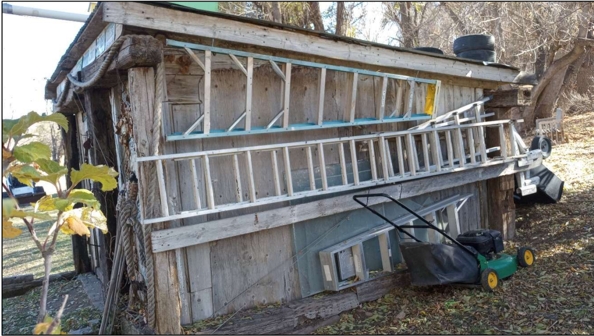
Site 5WL9807. The west elevation of Feature 5 (work shed), facing east. Photo by E. Garner, 11/19/2024.
