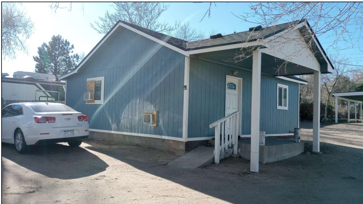
Site 5WL9808. The east and north elevations of Feature 3 (1999 residence), facing southwest. Photo by E. Garner, 11/19/2024.
