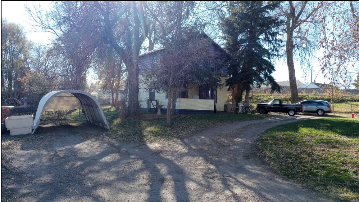
Site 5WL9807. Overview of the property from 5 th Street, facing southwest. Photo by E. Garner, 11/19/2024.
