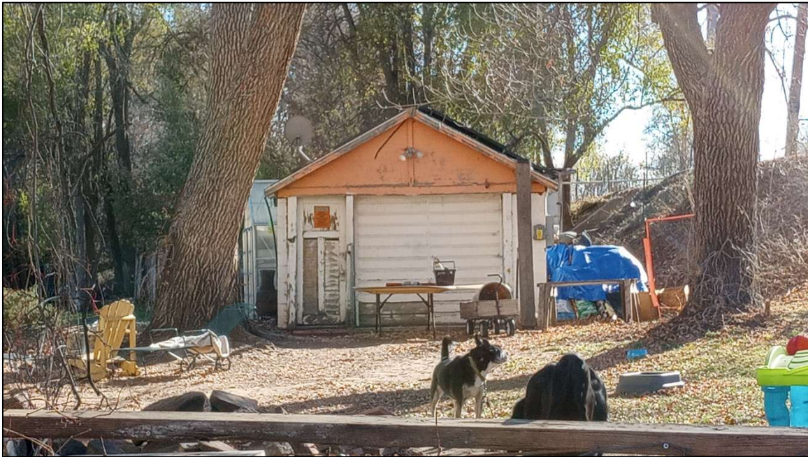
Site 5WL9807. The north elevation of Feature 2 (1952 garage), facing south. Photo by E. Garner, 11/19/2024.
