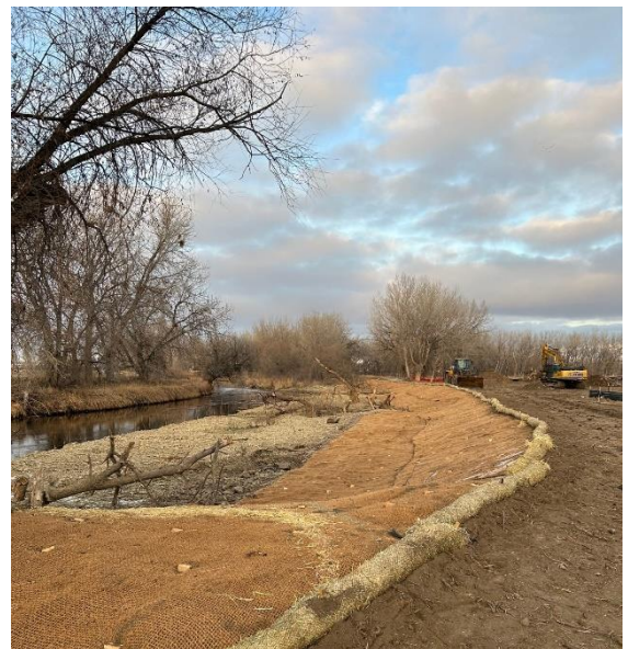
Riverbank improvements are completed on the Duran project, trail construction will be completed in January.
