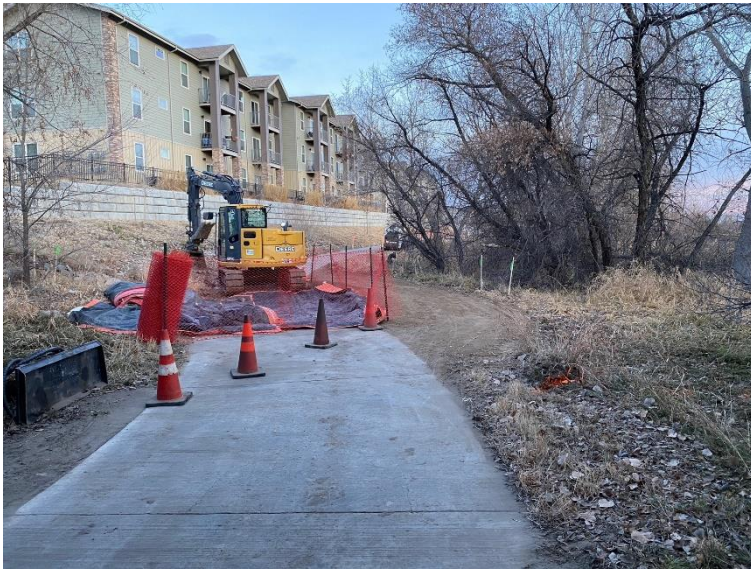
Work on the connector trail between the Sheep Draw Trail and the Pumpkin Ridge neighborhood.
