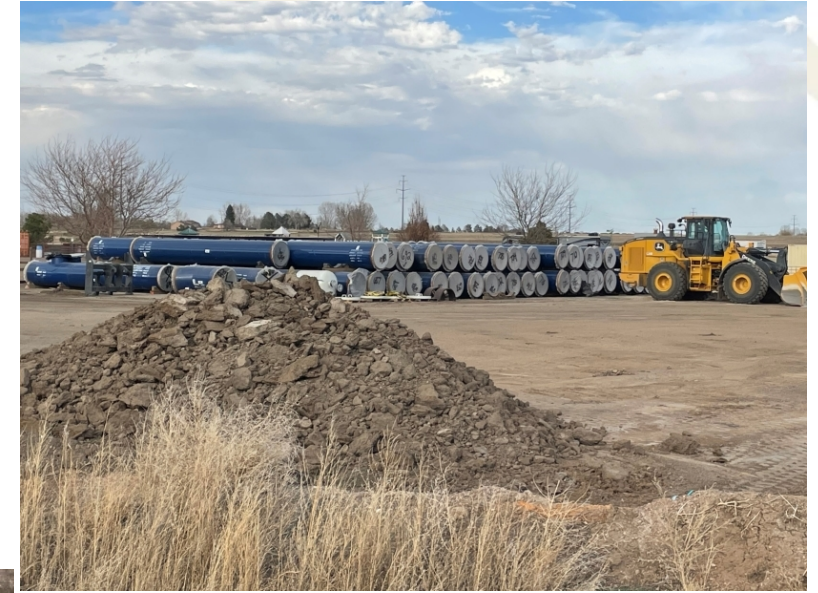
First loads of pipe
