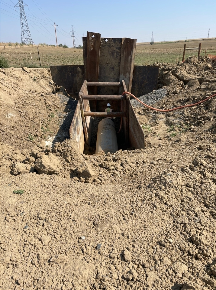
Bulkhead at end of Segment 1
