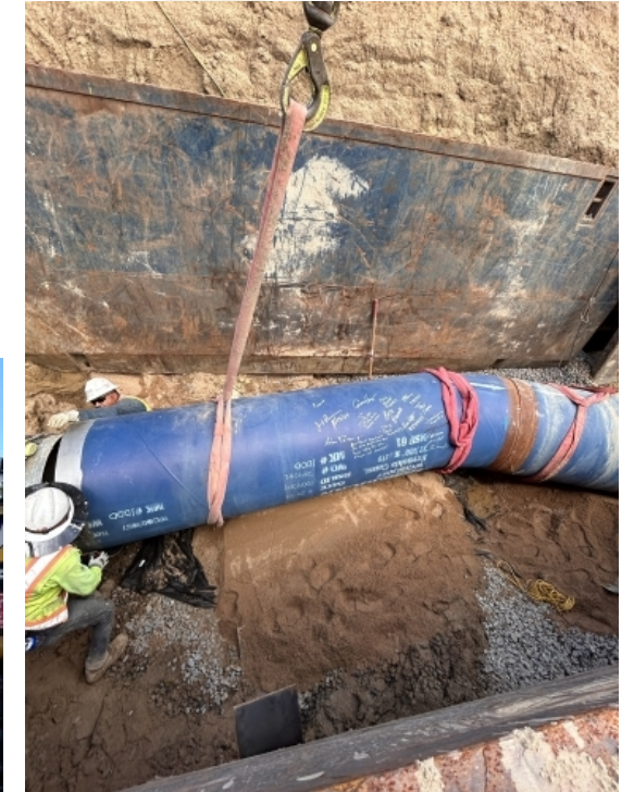
Setting last section of pipe
