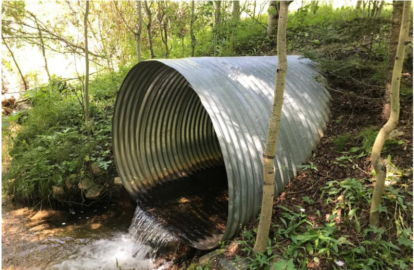
Perched culvert replaced with ford
