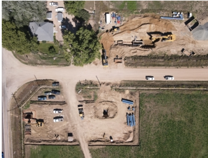
Laying pipe at SH 257 and CR 78
