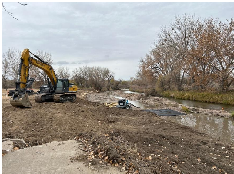
The repair of the Duran section of the Poudre River Trail, as seen in November. The coffer dam is in place and riprap placement is underway.
