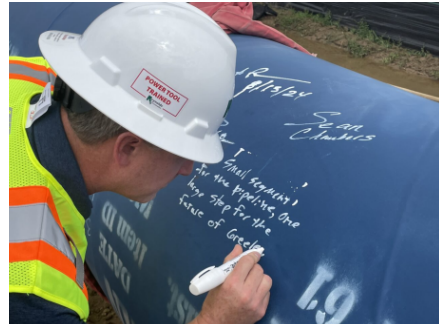
Terry Ranch Pipeline
