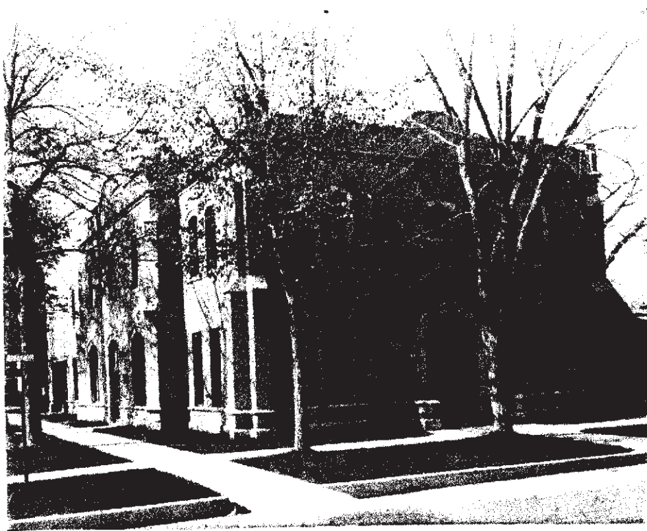
Exterior view of Allnutt Funeral Service – Macy Chapel, 702 13th St., Greeley. The building was constructed in 1918 and expanded in the 1960s. 101 years later, operations moved permanently to 6521 W. 20th St., Greeley. (Courtesy)
