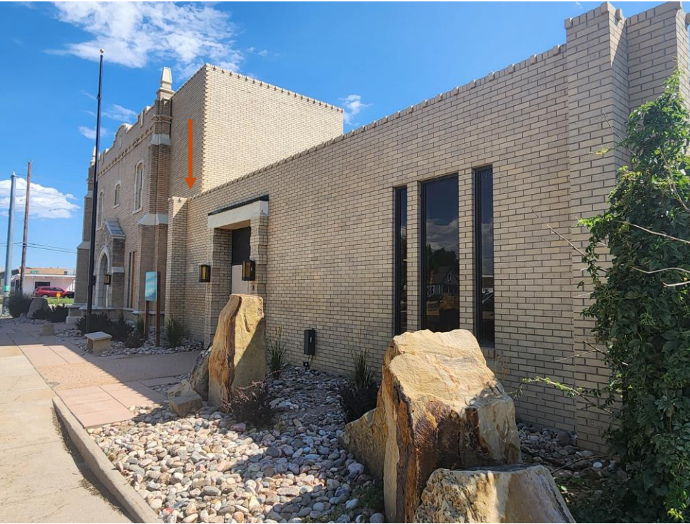
North view of addition; note interface of new bldg. with complementary matching brick
