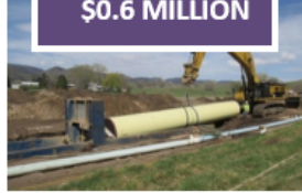
Bellvue Pipeline Goldhill Segment
