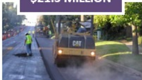
Pavement Rehabilitation & Concrete Repair
