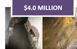
General Drainage System Repairs
