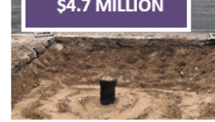
Distribution Pipeline Replacement
