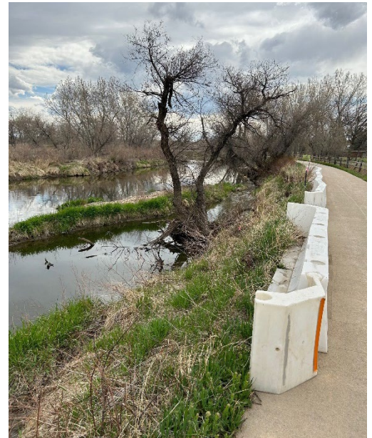
The Duran section of the Poudre Trail, with a view of the trail before the repair project began.
