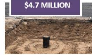
Distribution Pipeline Replacement
