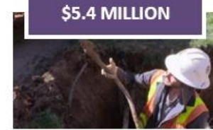
Lead Service Line Replacement
