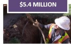
Lead Service Line Replacement
