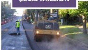
Pavement Rehabilitation & Concrete Repair
