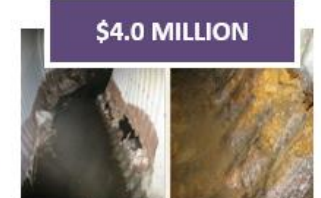
General Drainage System Repairs
