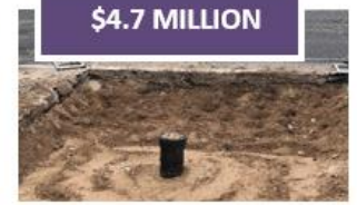
Distribution Pipeline Replacement
