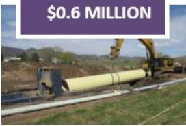
Bellvue Pipeline Goldhill Segment
