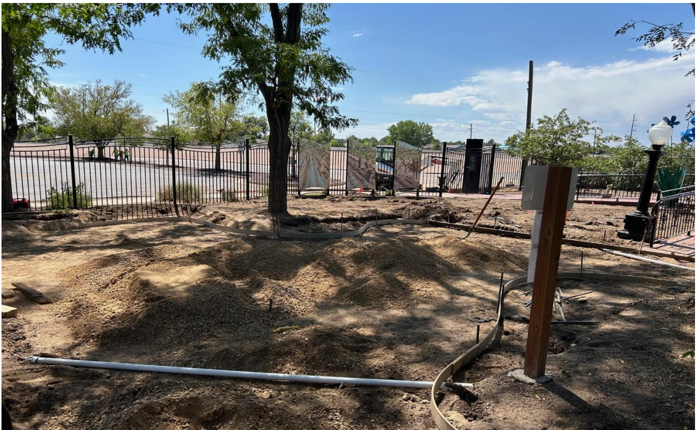
Excavation for new concrete entry patio
