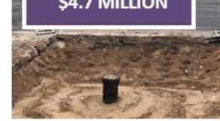
Distribution Pipeline Replacement
