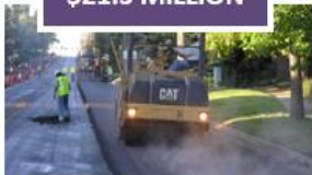
Pavement Rehabilitation & Concrete Repair
