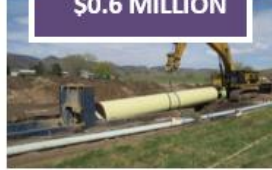
Bellvue Pipeline Goldhill Segment
