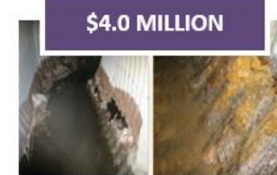
General Drainage System Repairs
