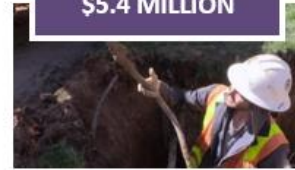
Lead Service Line Replacement
