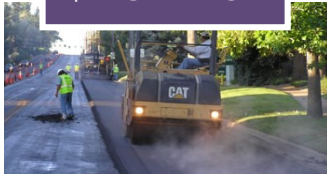
Pavement Rehabilitation, Concrete Repair, Cross-Pan Replacement
