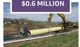
Bellvue Pipeline Goldhill Segment
