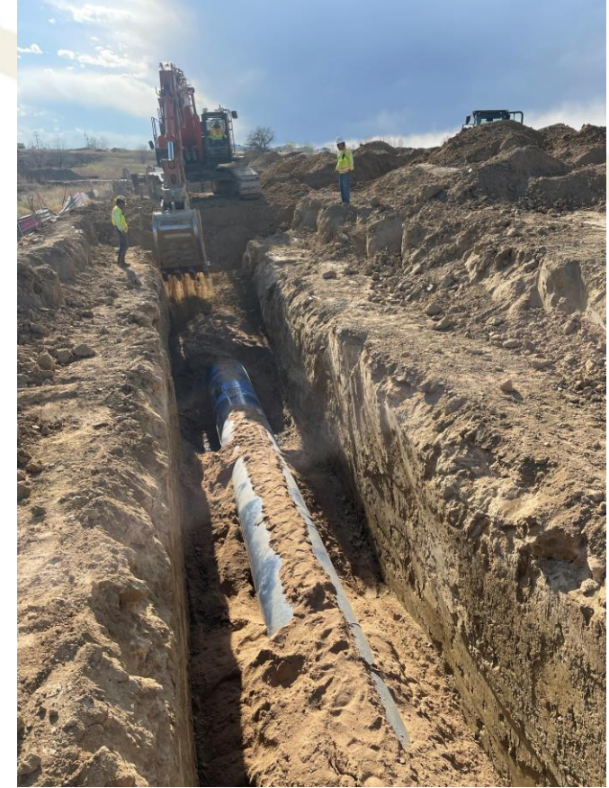
Bedding and covering pipe
