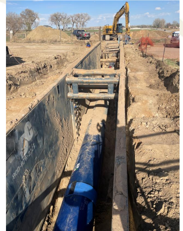
Laying pipe at Hwy 14 and CR 19
