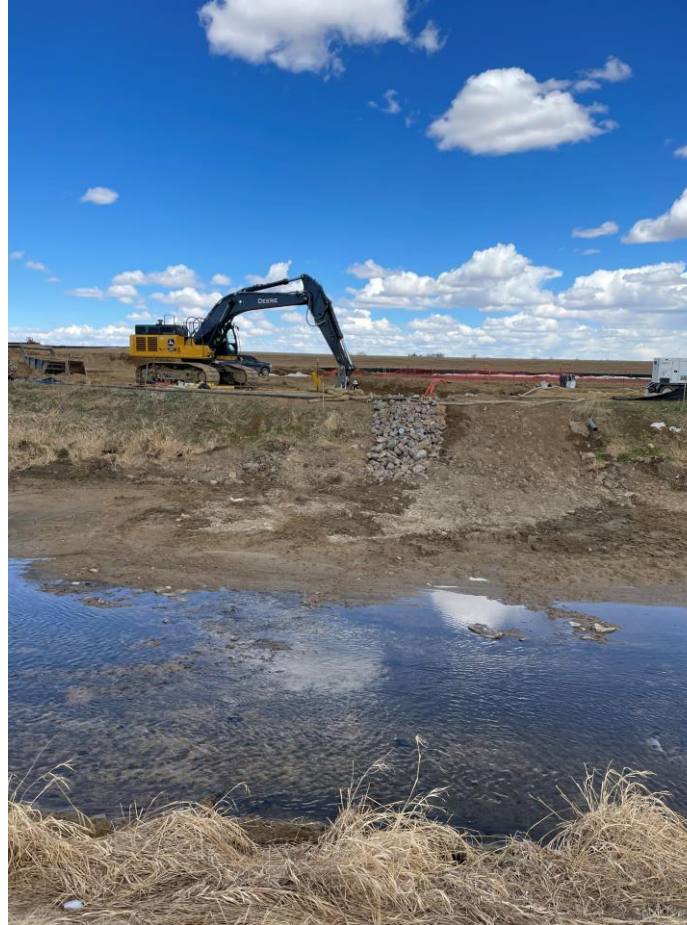
Installing blowoff at LWIC
