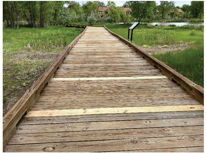
Repairs to warped and cracking sections of the boardwalks at Signature Bluffs NA were replaced in May.
