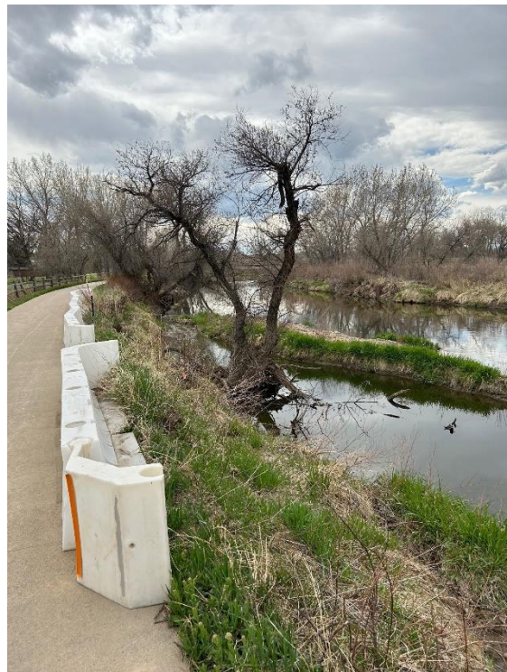
View upstream at PRT Duran section.
