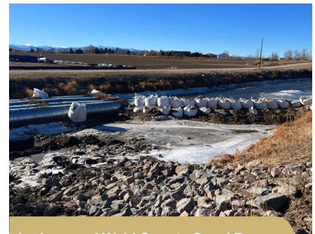
Larimer and Weld County Canal Bypass
