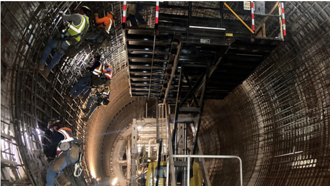
Crews place rebar along the tunnel's inner walls, necessary to reinforce the concrete liner.
