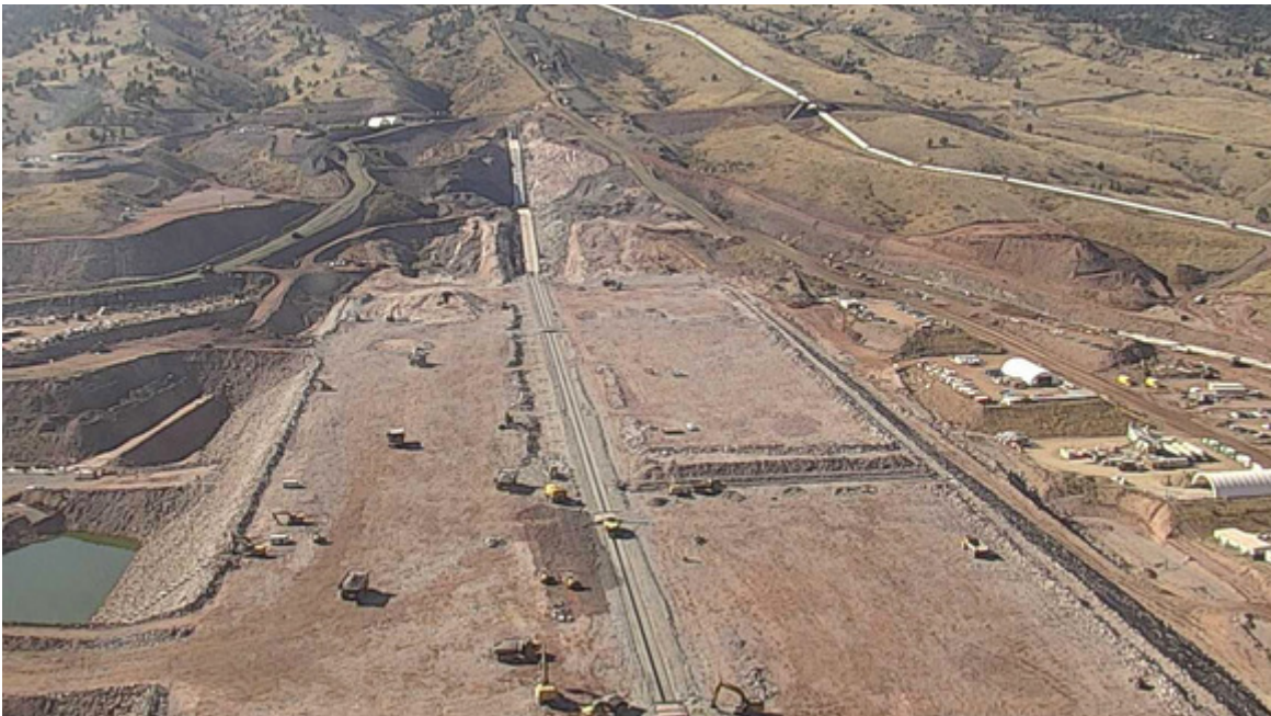
A trench was recently dug across the main dam to place sensitive equipment for monitoring the dam safety.
