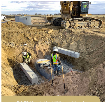
CARV Install at Winter North
