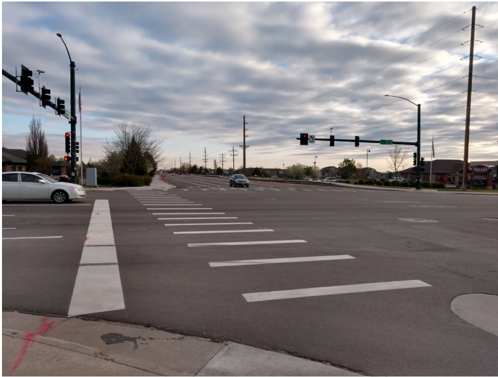
20 th Street and 71 st Ave Looking North
