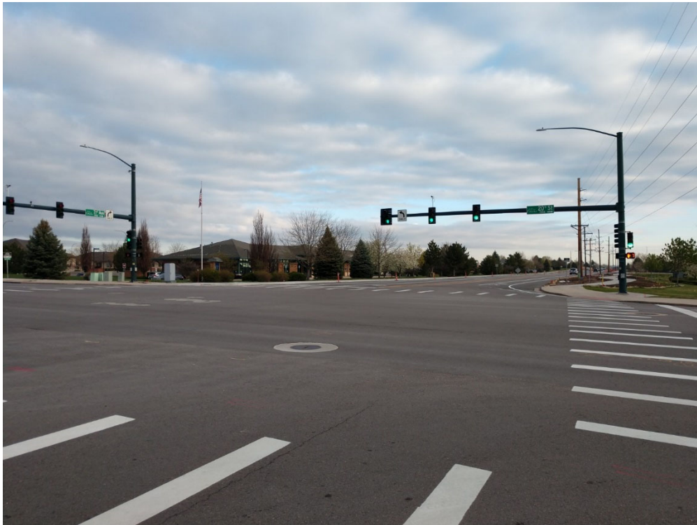
20 th Street and 71 st Ave Looking North
