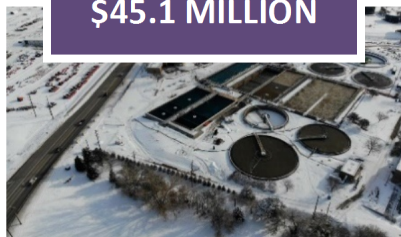
Wastewater Treatment Reclamation Facility (WTRF) Phase 2
