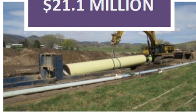
Bellvue Pipeline - Gold Hill Segment
