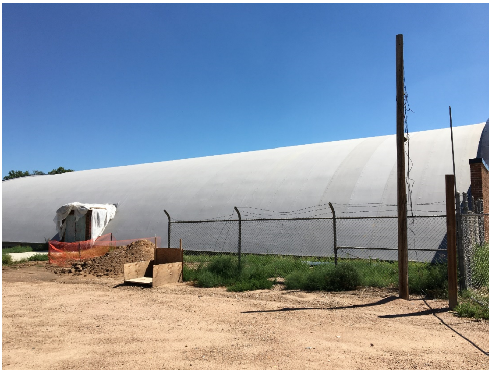
West façade, looking east-northeast
