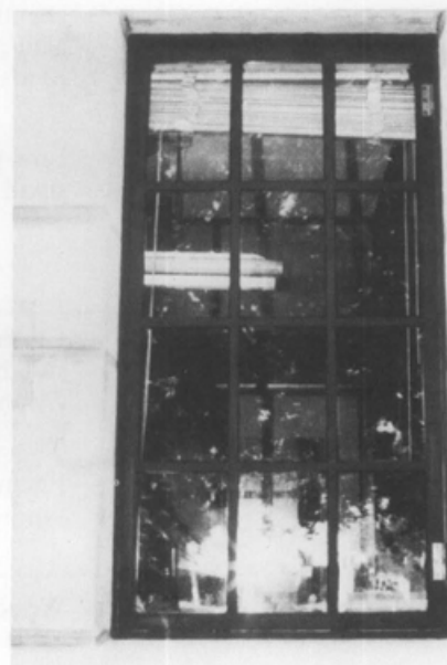
Fig. 6 d. View looking down towards the sill. The subframes appeared very rusted, but were in good condition once debris was vacuumed and surface rust was removed, in place, with chemical compounds. Where necessary, epoxy and steel filler was used to patch depressions in order to make the subframe serviceable again.
