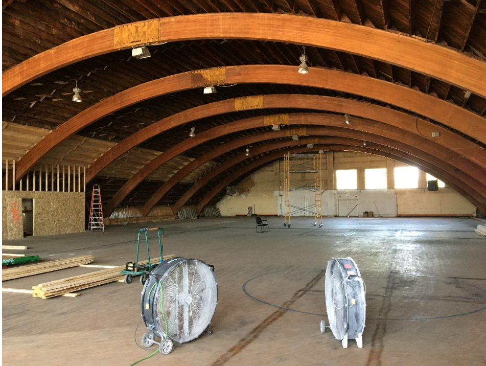
Interior, looking north
