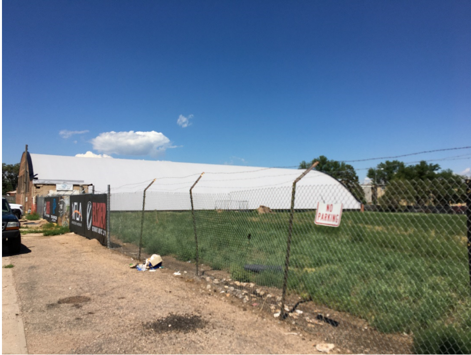
East façade, looking west
