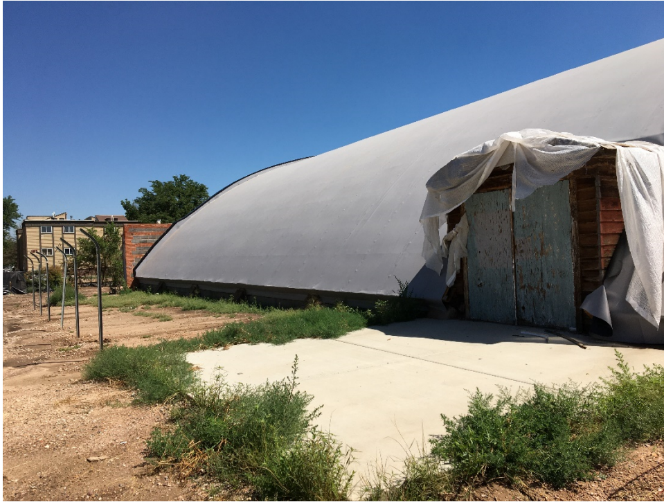
West façade looking north-northeast
