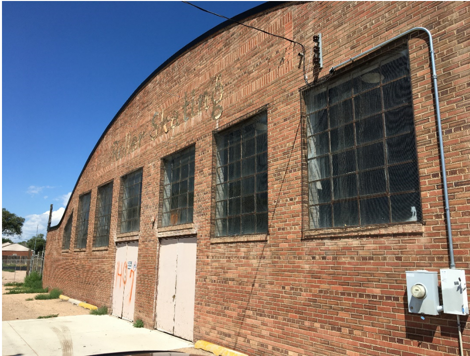
South façade, looking northwest
