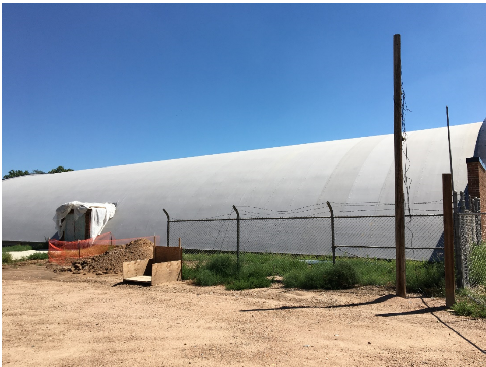
West façade, looking east-northeast
