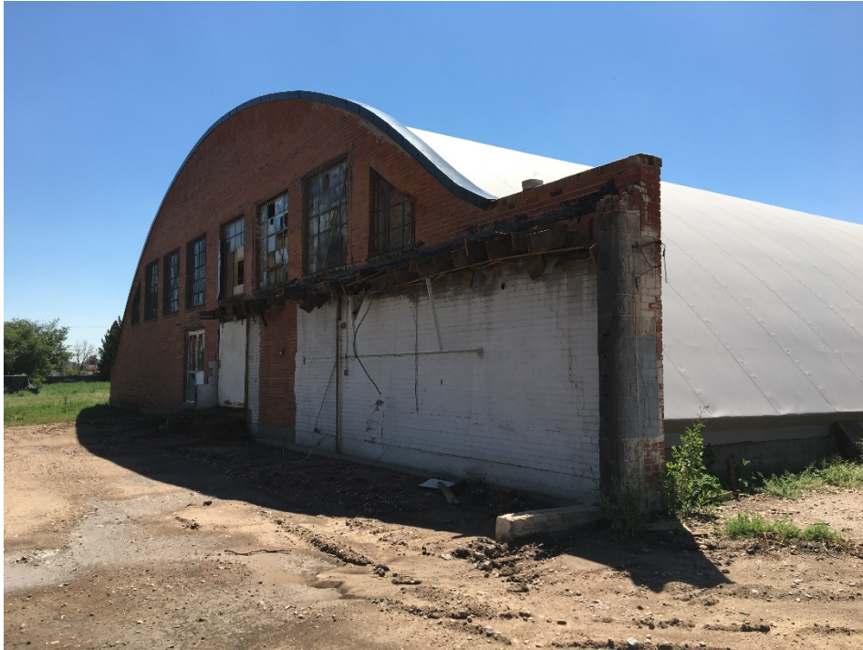
North façade, looking southeast
