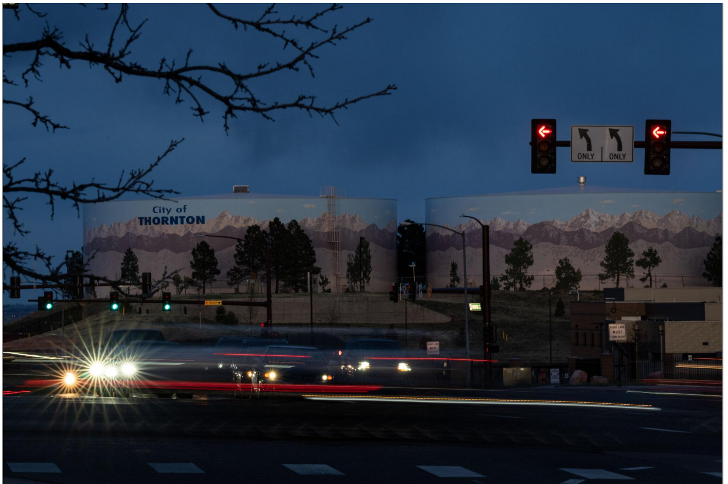
The Thornton water treatment plant.
