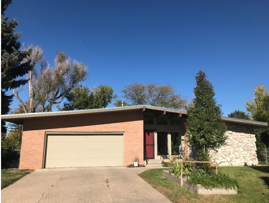
South elevation, Photo by Linde Thompson, October 2021.
