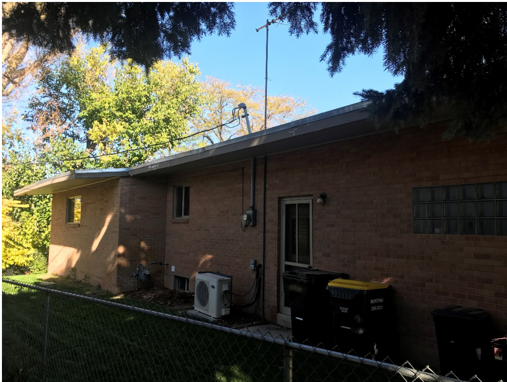
West elevation, Photo by Linde Thompson, October 2021
