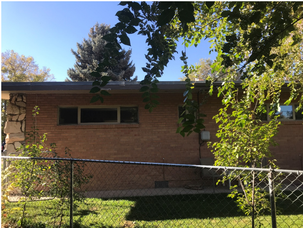
East elevation, Photo by Linde Thompson, October 2021.
