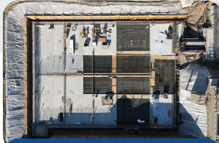
Selector Basins 1 & 2 Concrete and Rebar
