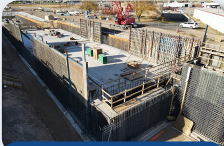
Aeration Basin 0 Wall Forms and Rebar
