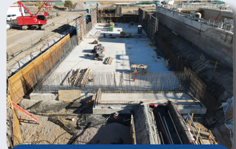
Aeration Basin 0 Slab Concrete
