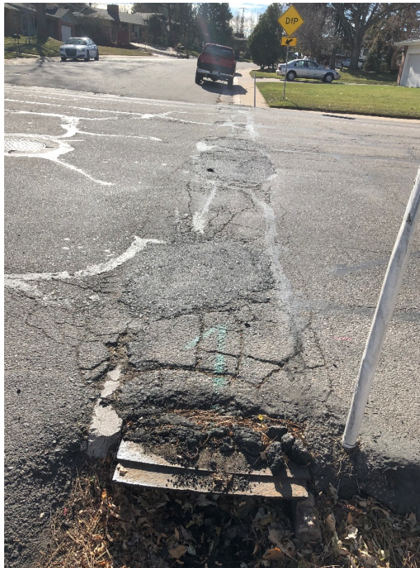
20 th St Culvert
