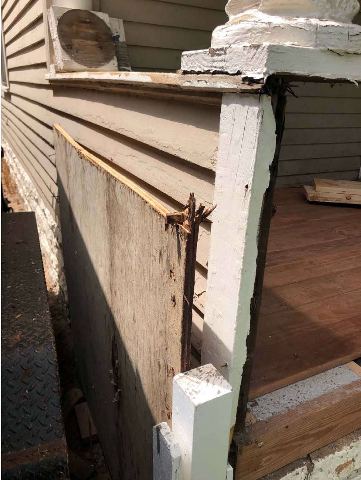
South side of porch not in need of repair (this is how the porch originally looked on the north and it will be returned to this on the north).
