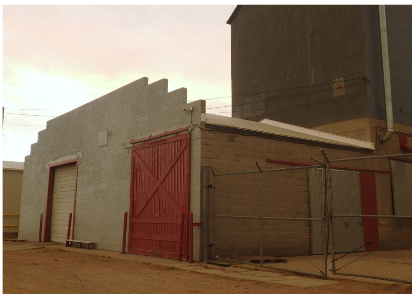
Figure 79. 608 9th Street. Building located along 8th Avenue side of parcel. This industrial warehouse constructed from CMUs shows the use of a false front to hide a gable roof.
