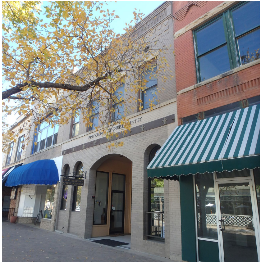
Figure 77. The Bijou Theatre, 826 9th Street (5WL.4155). Although the ground story of this 1906 building has been altered, it retains the basic elements of a Two-Part Commercial Block with a public entry for commercial—or in this case religious—use and upper stories for offices or other private functions. Although constructed at the beginning of the 20th century, this building is an example of the late-19th century commercial style with its restrained ornamentation and decorative brickwork.
