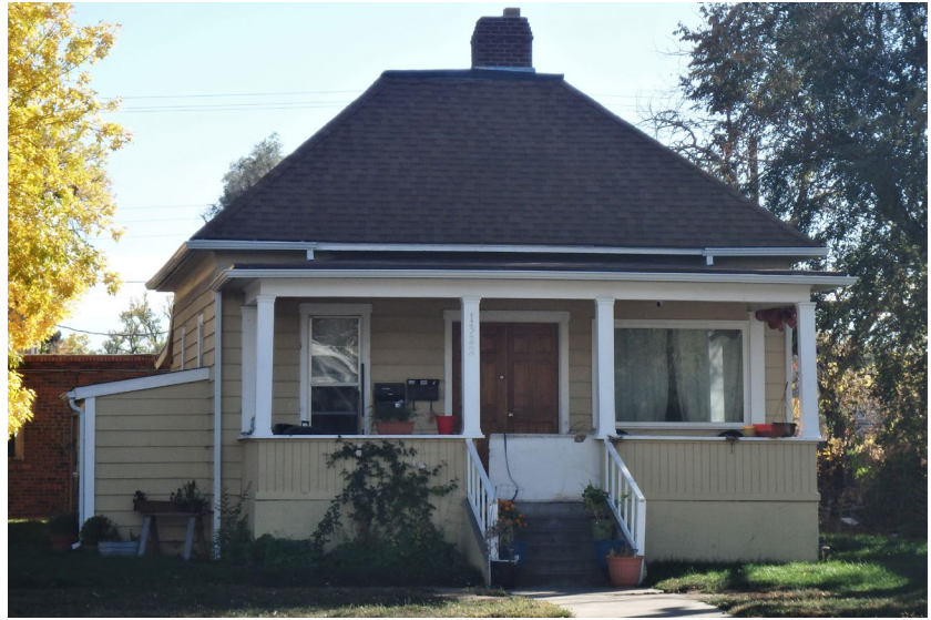
Figure 84. 1322 8th Street. This Hipped-Roof Box house is characterized by its hipped roof and full-width front porch. There are many examples of this form in Greeley. This residence possesses a truncated roof and lacks a dormer window.
