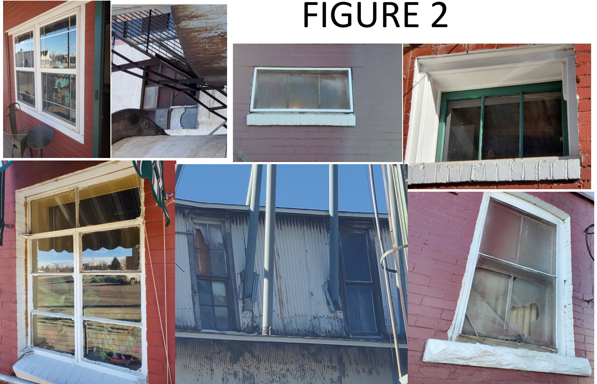
A panoply of existing window styles. Clockwise from upper left corner: 6 lite prairie grid vinyl windows, large colonial-grid style window, 3 lite steel windows, 3 lite wood windows , 2 lite double hungwood window. 4, 2, and 1 lite single hung wood windows, and 4 lite steel casement windows, There is an additional colonial-grid style window in the garage, which is boarded up and impossible to access for photography purposes..
