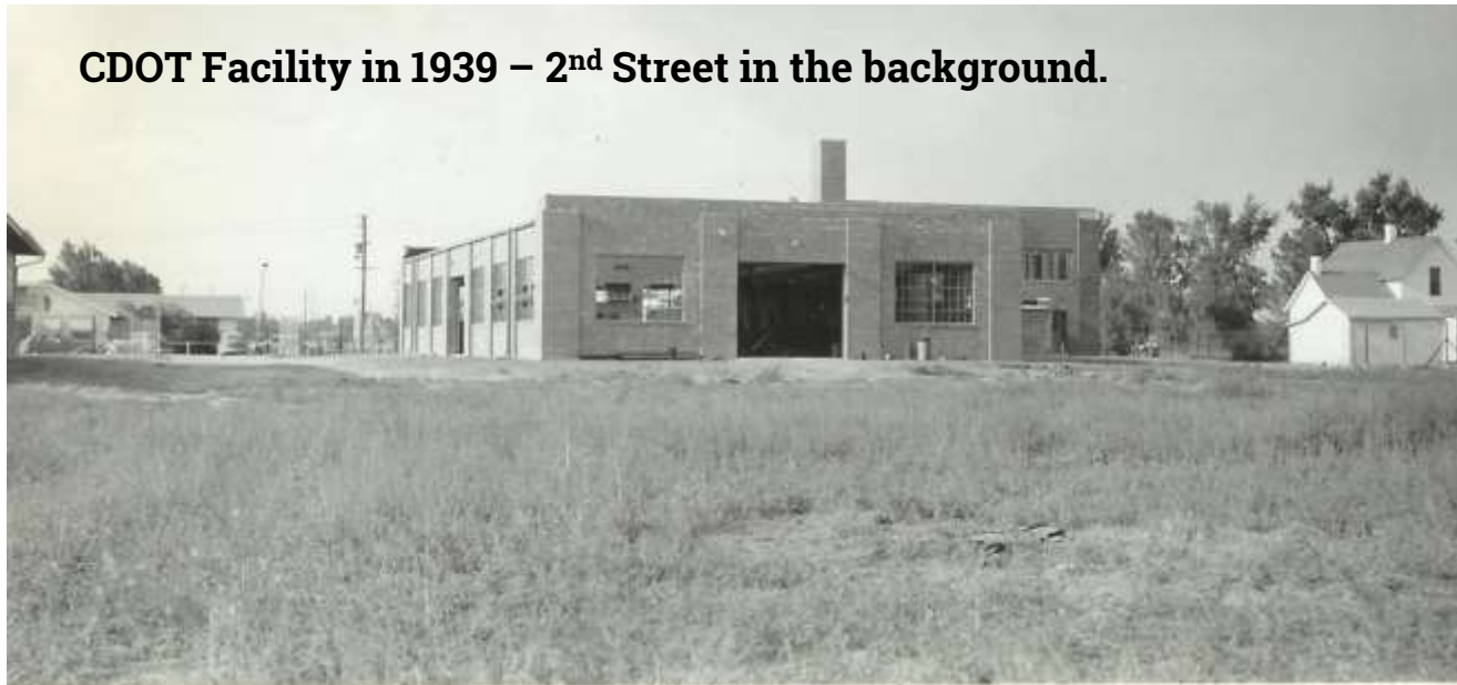
REELEY, WEST AND SOUTH FRONT OF SHOP.
