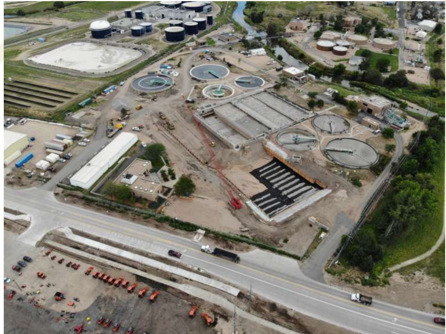
Greeley WTRF Construction Progress as of August 23, 2021
