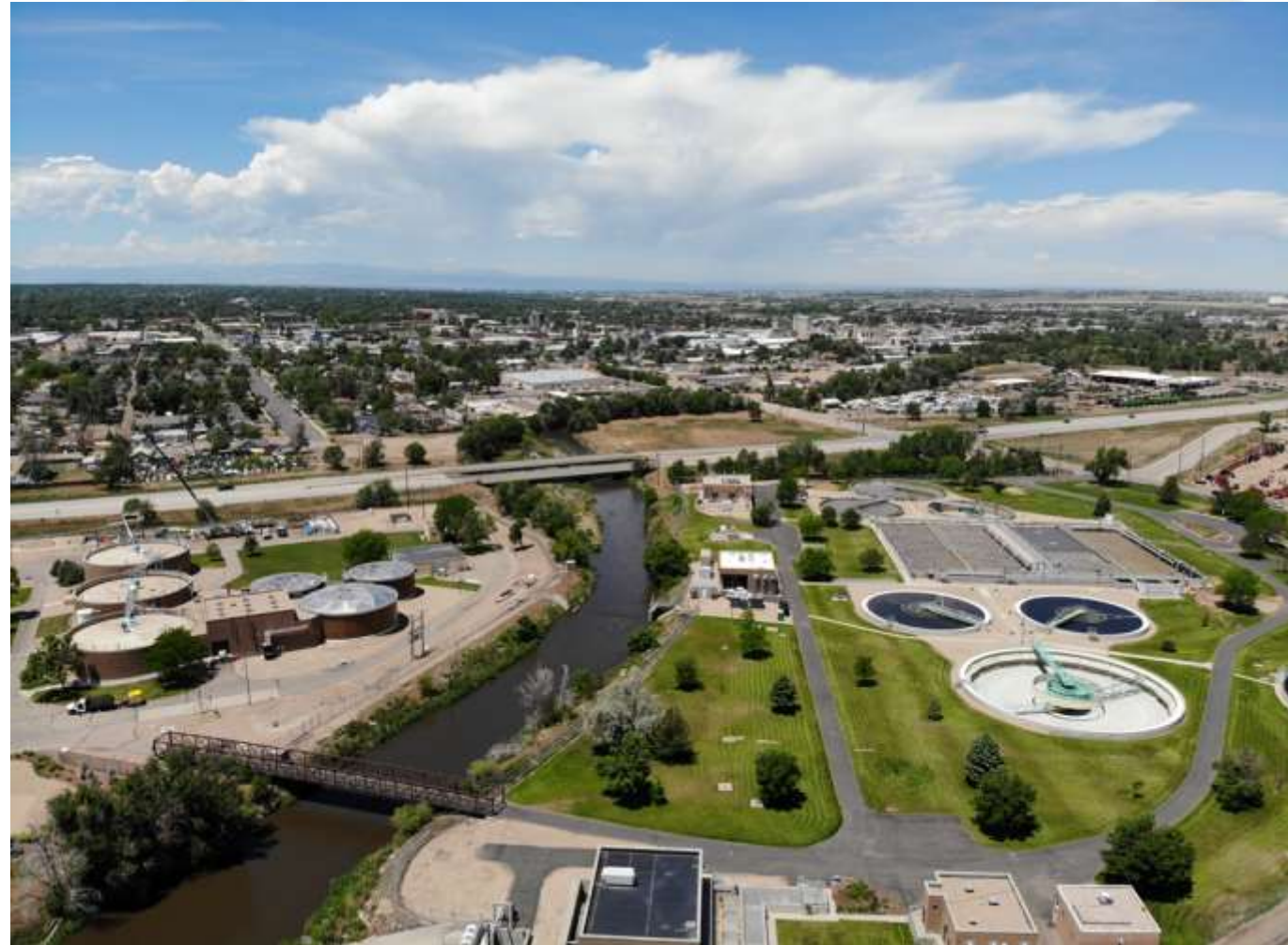
City of Greeley Wastewater Treatment & Reclamation Facility - Pre-Construction
