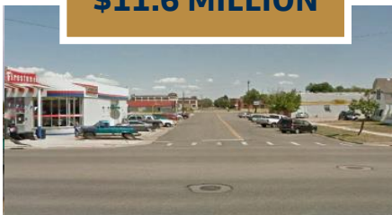
12th Street Storm Trunk Line - Phase 1B
