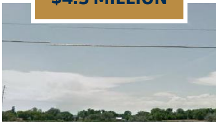
12th Street Storm Trunk Line - Phase 1A
