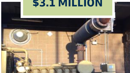
Wastewater Treatment & Reclamation Facility (WTRF) Generator Replacement
