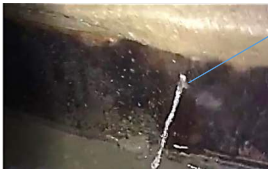
Figure 2.4: FM 7 site infiltration runner along manhole channel
