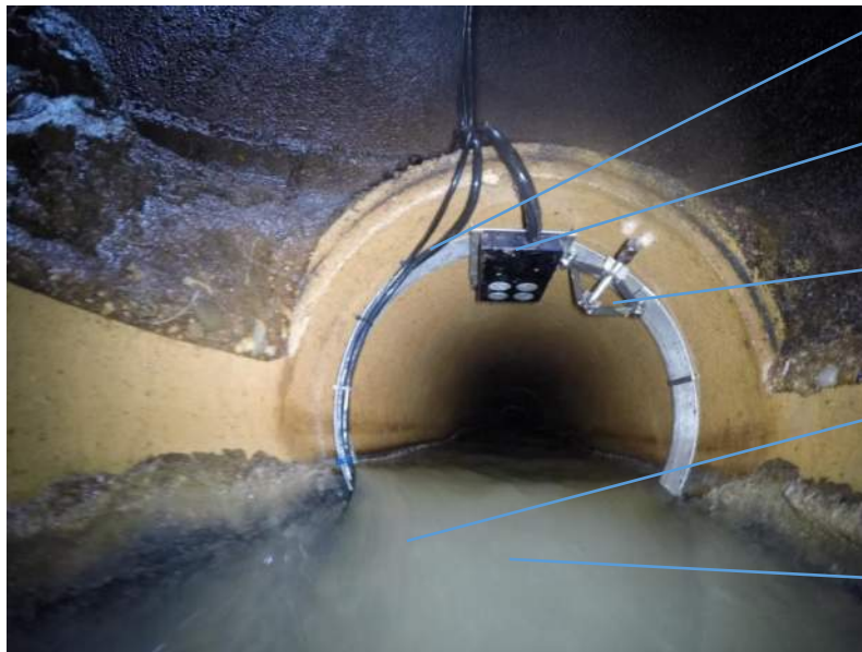
Figure 2.2: FM 03 Flow Meter Installation
